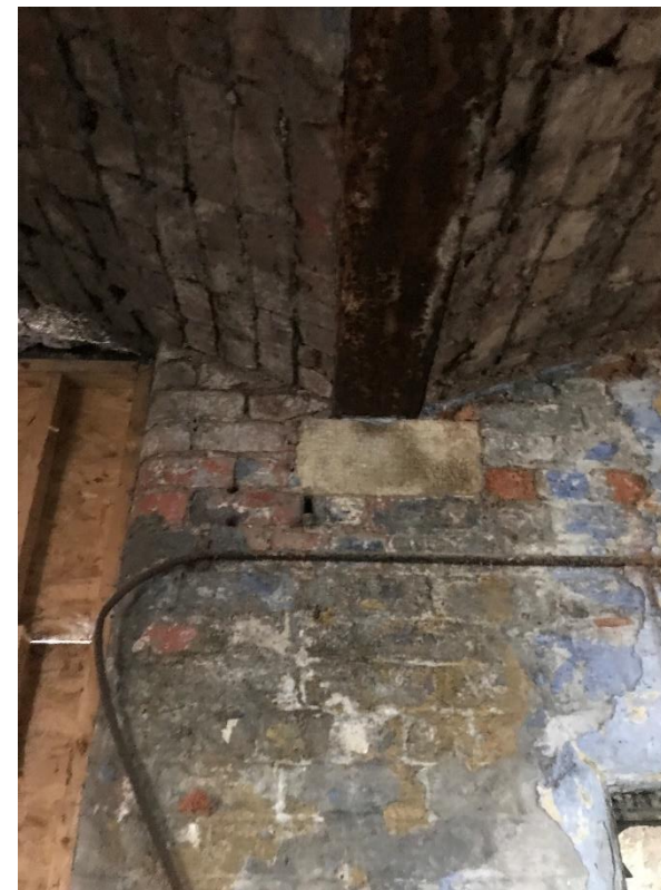
Figure 5: Padstone supporting structural beam.
