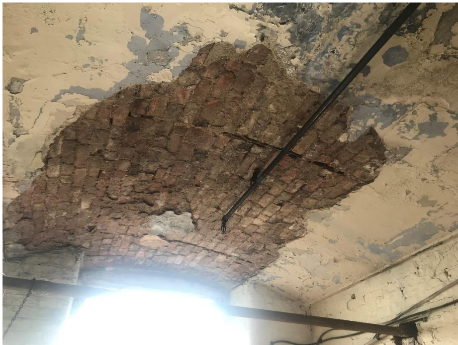
Figure 2: Thrust Tie Bars in Masonry Jack Arch
