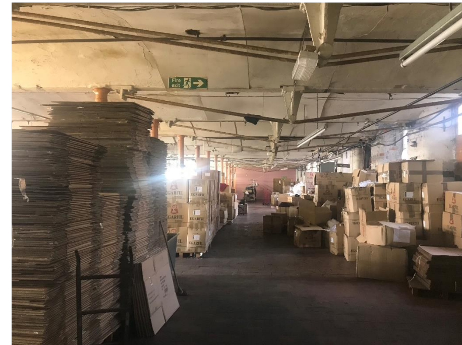
Figure 1: Masonry Jack Arch Floor Slabs on Cast Iron Frame
