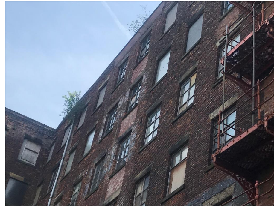
Figure 4: External Solid Masonry Walls
