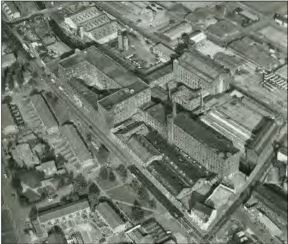
Plate 10: Aerial view of Brunswick Mill and Pooley's Mill in the mid-1980s
