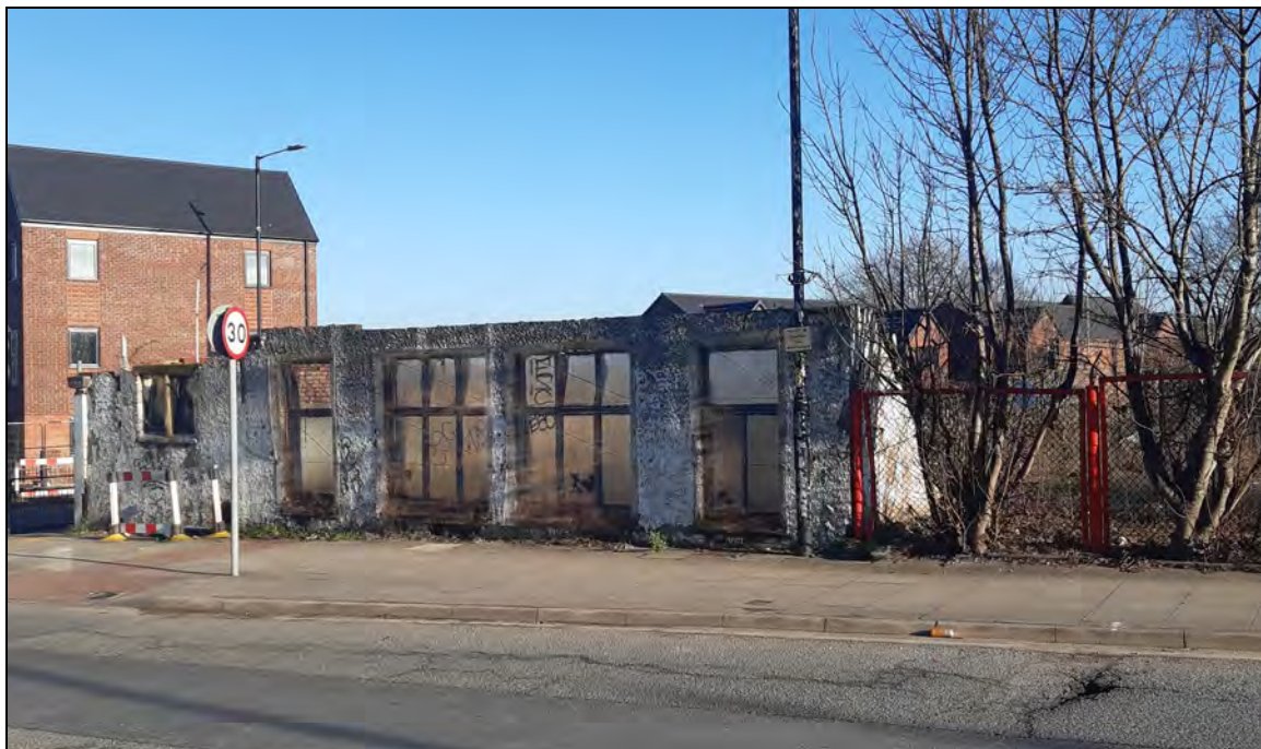
Plate 13: The demolished remains of the buildings occupying the Beswick Street frontage
