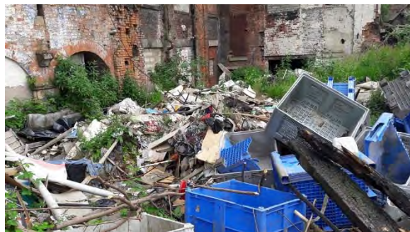
Photograph 5 (P5) Significant quantity of flytipped waste on open ground to the south of the mill building.
