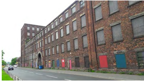
Photograph 1 (P1) View of Brunswick Mill building from Bradford Road.
