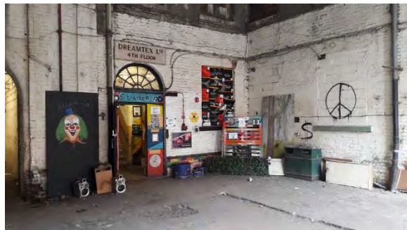
Photograph 3 (P3) Mill building currently used by contemporary commercial premises.
