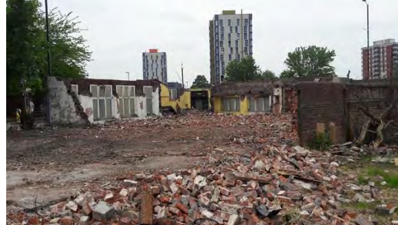
Photograph 8 (P8) Demolition rubble in area of former Methodist chapel.
