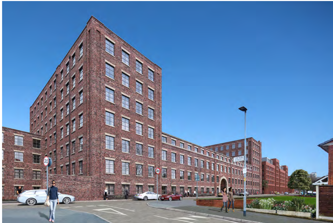
View south along Bradford Road of existing mill with new-build development in the background
