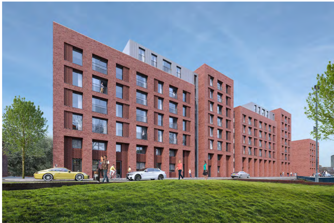
View south along Bradford Road of new-build intermediate block
