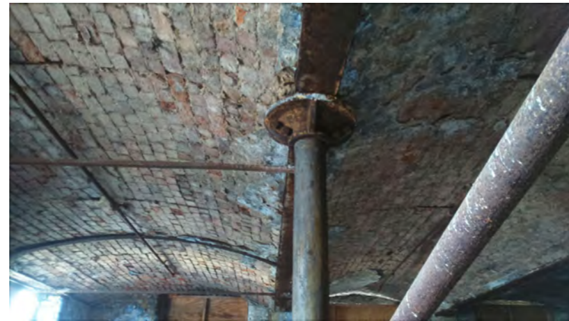
Existing mill floor structure
