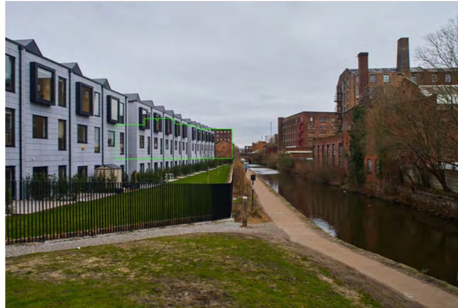
Verified View: VVP-04
