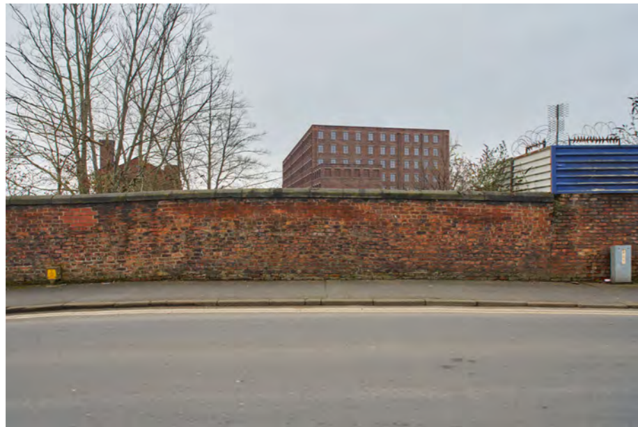
Verified View: VVP-05
