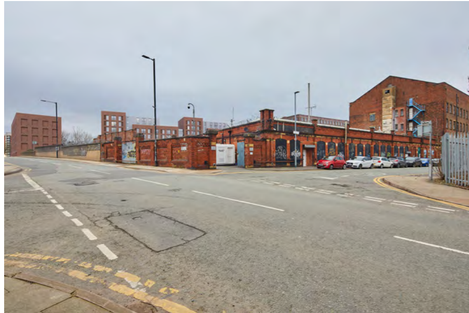
Verified View: VVP-01
