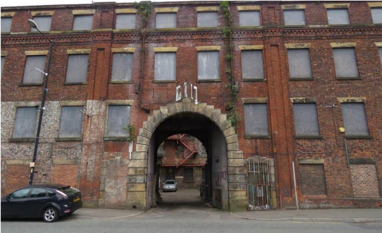
Figure 2.1: North front of the mill illustrating blocked up windows
