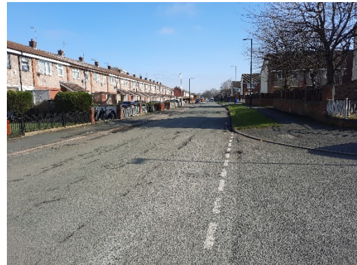
Photograph 14: View to the northeast along Ridgway Street.
