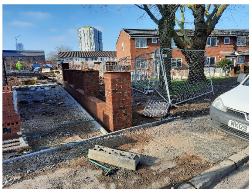
Photograph 15: Ongoing construction work on Halmore Road.
