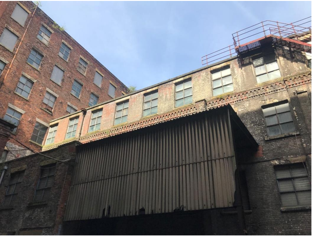
Figure 78: External Steel Lean to Canopy Installed
