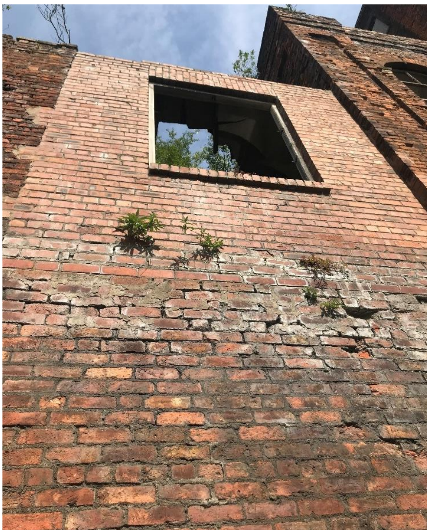
Figure 71: Reconstructed Boiler House Wall
