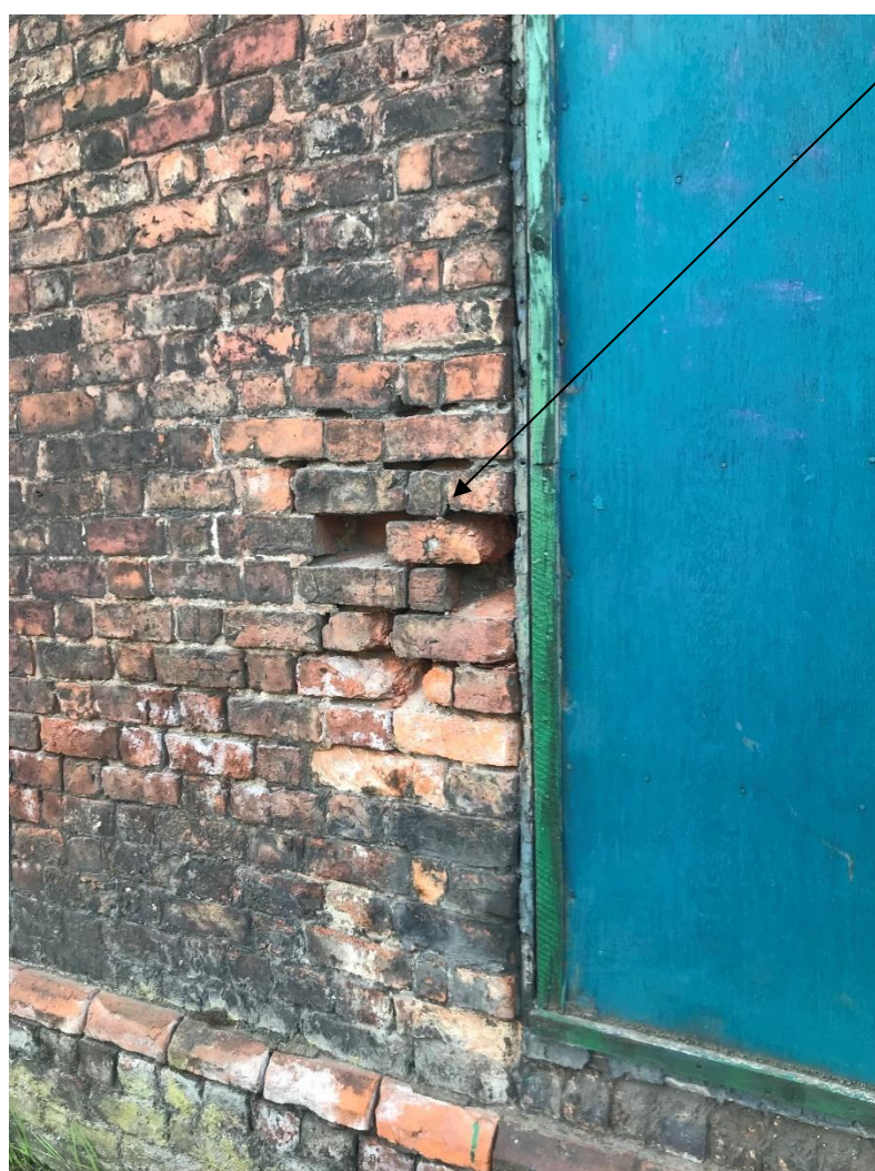
Figure 64: General Loss of Masonry and Pointing
