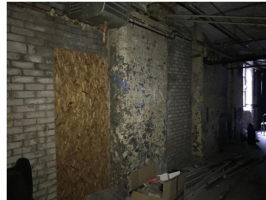
Figure 53: Infilled Openings
