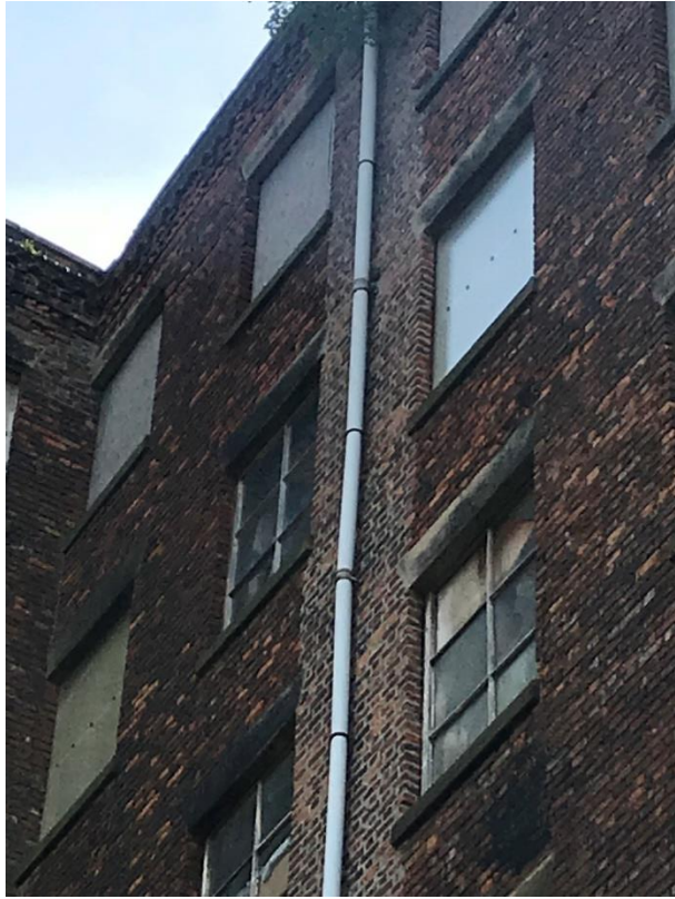
Figure 86 Repointed Brickwork
