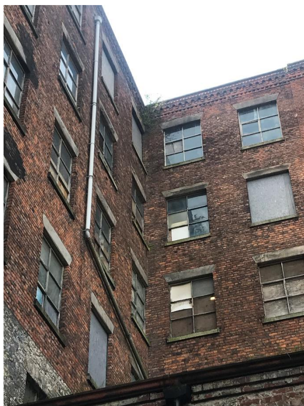
Figure 91: Opening Line Corresponding with Wing Interface Line
