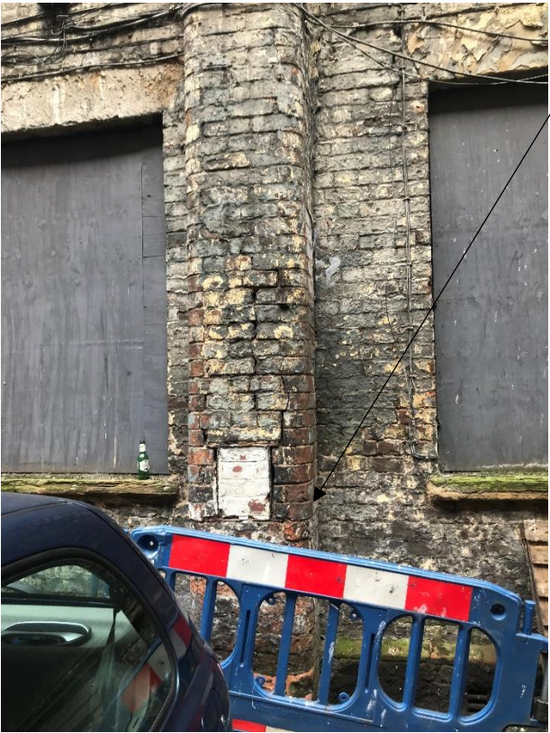
Figure 80: Steel Beam Ends Built into Masonry Pier
