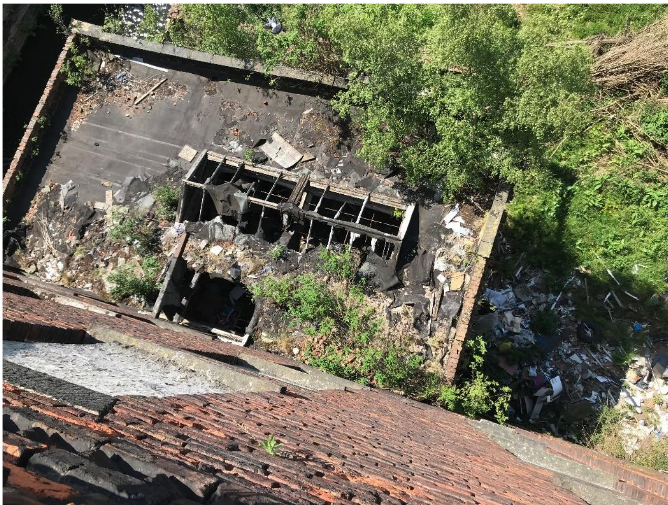
Figure 12: Boiler House Roof Looking Down from Mill Roof
