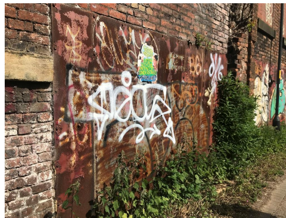
Figure 72: Infill to Historic Openings
