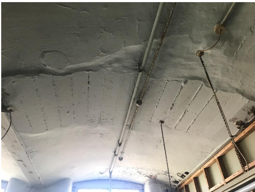
Figure 28: Concrete Patch Repair to Arch Soffit
