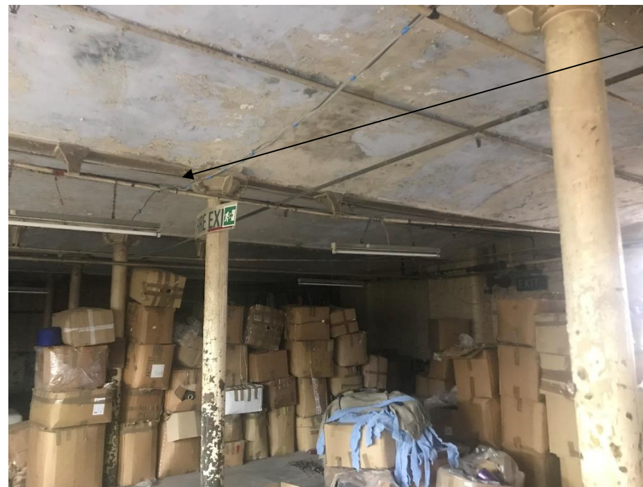
Figure 50: Lateral Tie Bar South Eastern Wing
