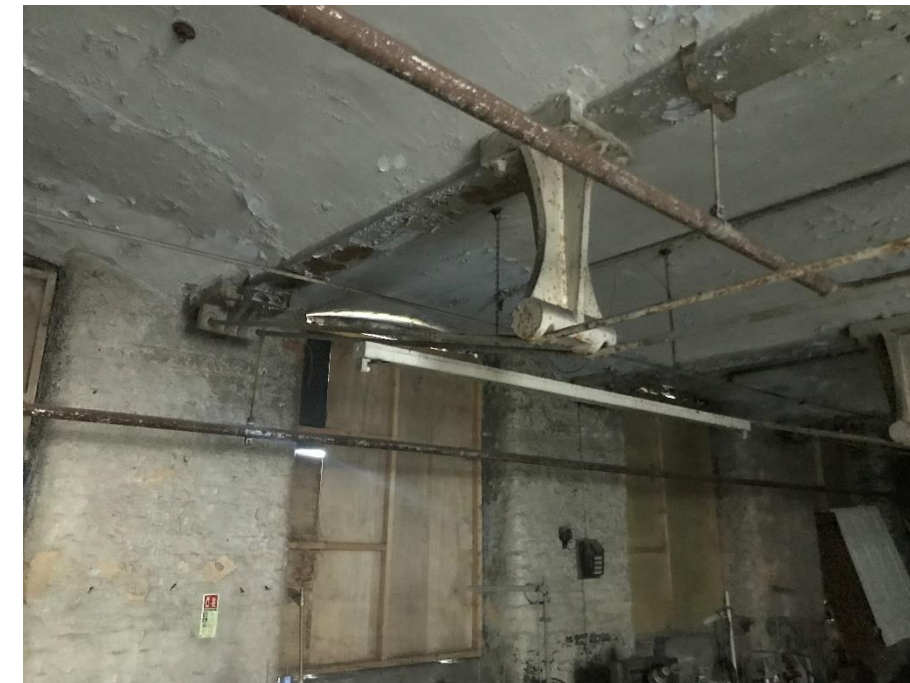
Figure 52: Beam Strengthening.
