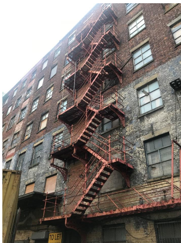
Figure 90: Historic Staircase and Associated Openings Infilled with Engineering Brick
