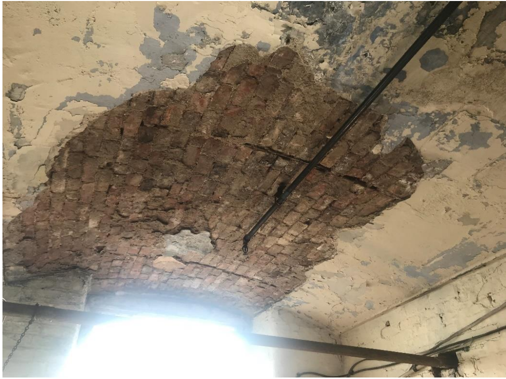
Figure 6: Thrust Tie Bars in Masonry Jack Arch
