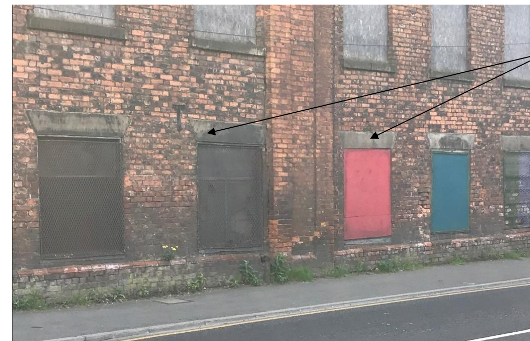
Figure 63: Damaged Masonry Pier and Associated Lintels
