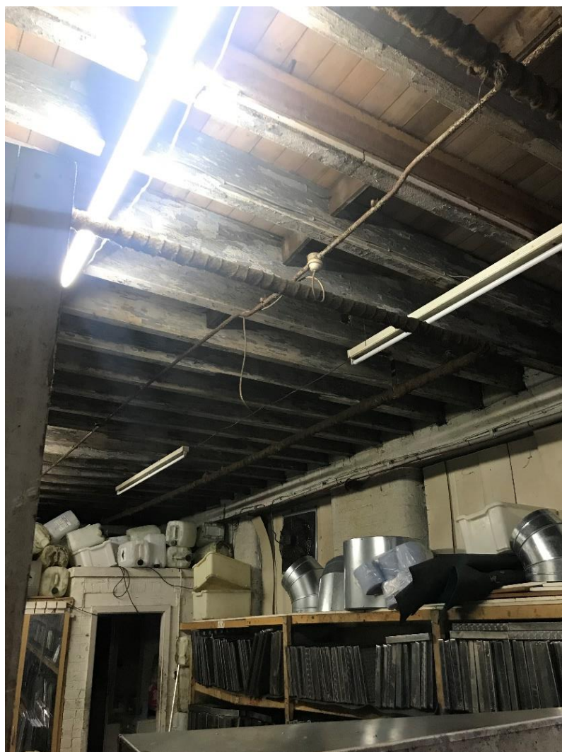
Figure 54: Two Storey Courtyard Building. First Floor Timber Construction Observed from Ground
