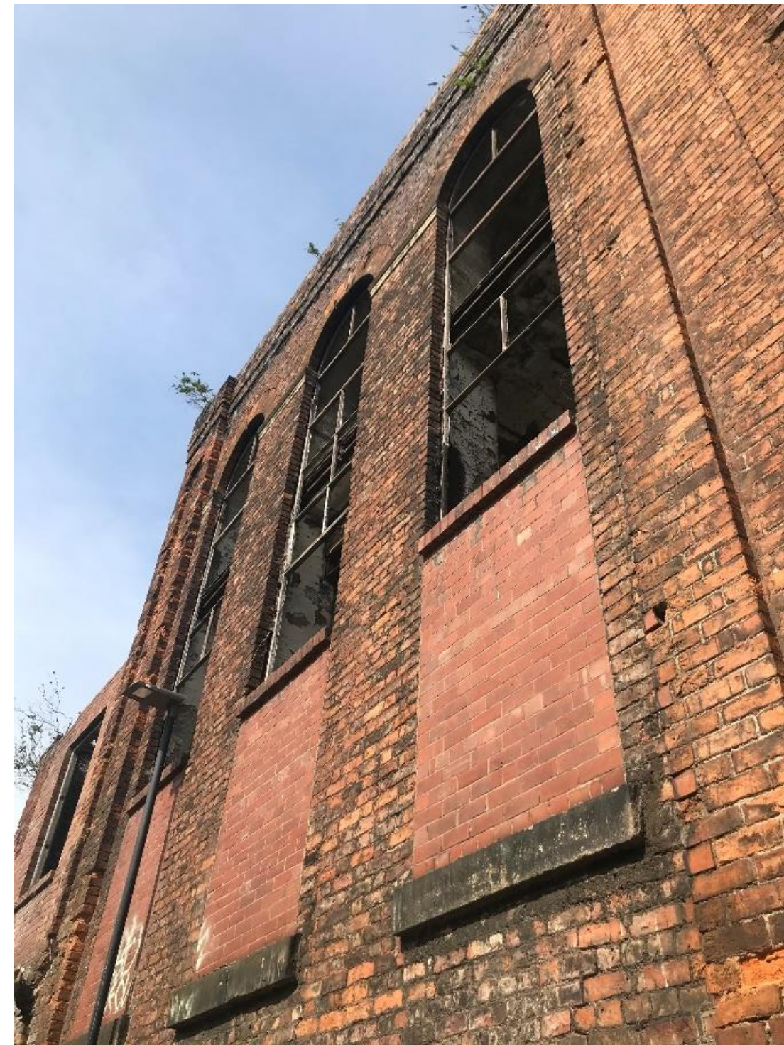
Figure 13: Rear Elevation of Boiler House from Towpath
