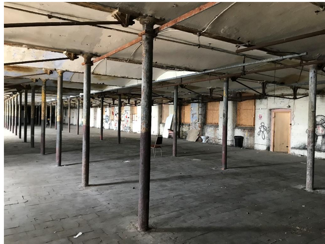
Figure 38: Strengthened Inner and Outer Bays
