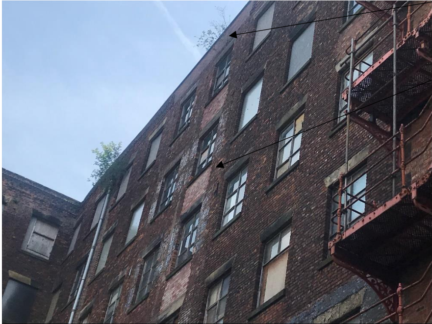
Figure 88 Infilled Openings to Southern End of Elevation 7
