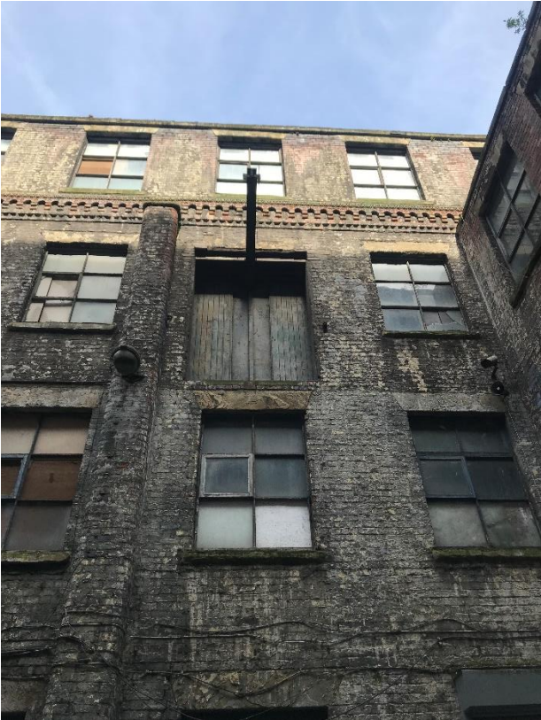
Figure 81: High Level Beam Coinciding with Beams Below. Possible Former Hoist
