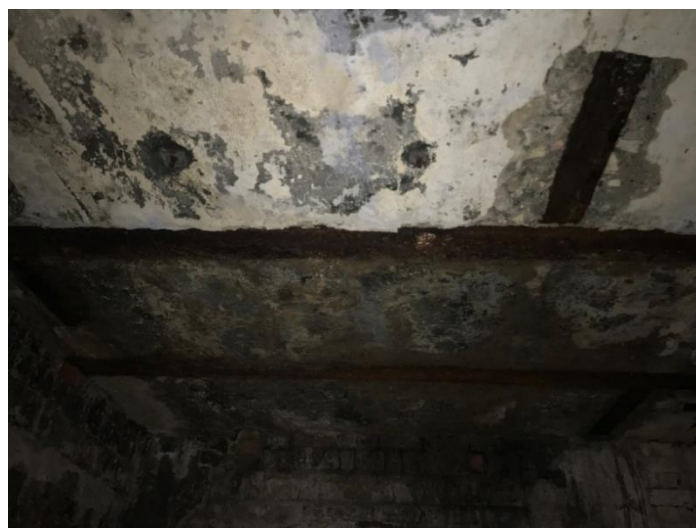
Figure 9: Steel Filler Joist Floor
