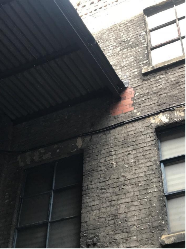
Figure 79: Engineering Brick Supporting Steelwork
