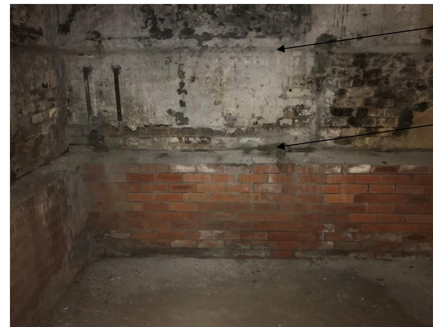
Figure 60: Corbelled Walls
