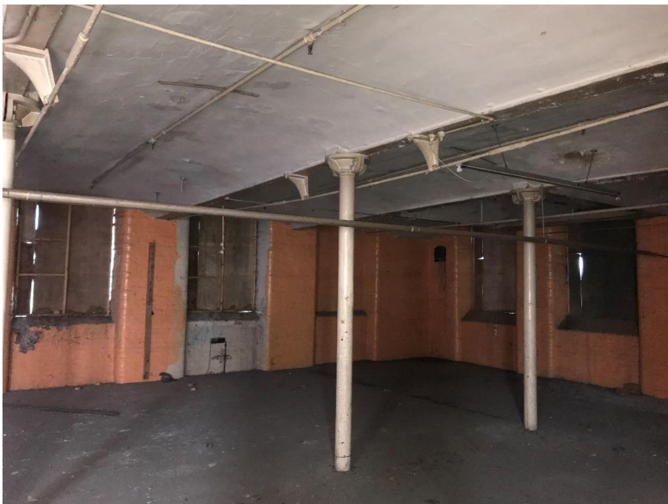
Figure 37: Lateral Tie Bars Between Piers
