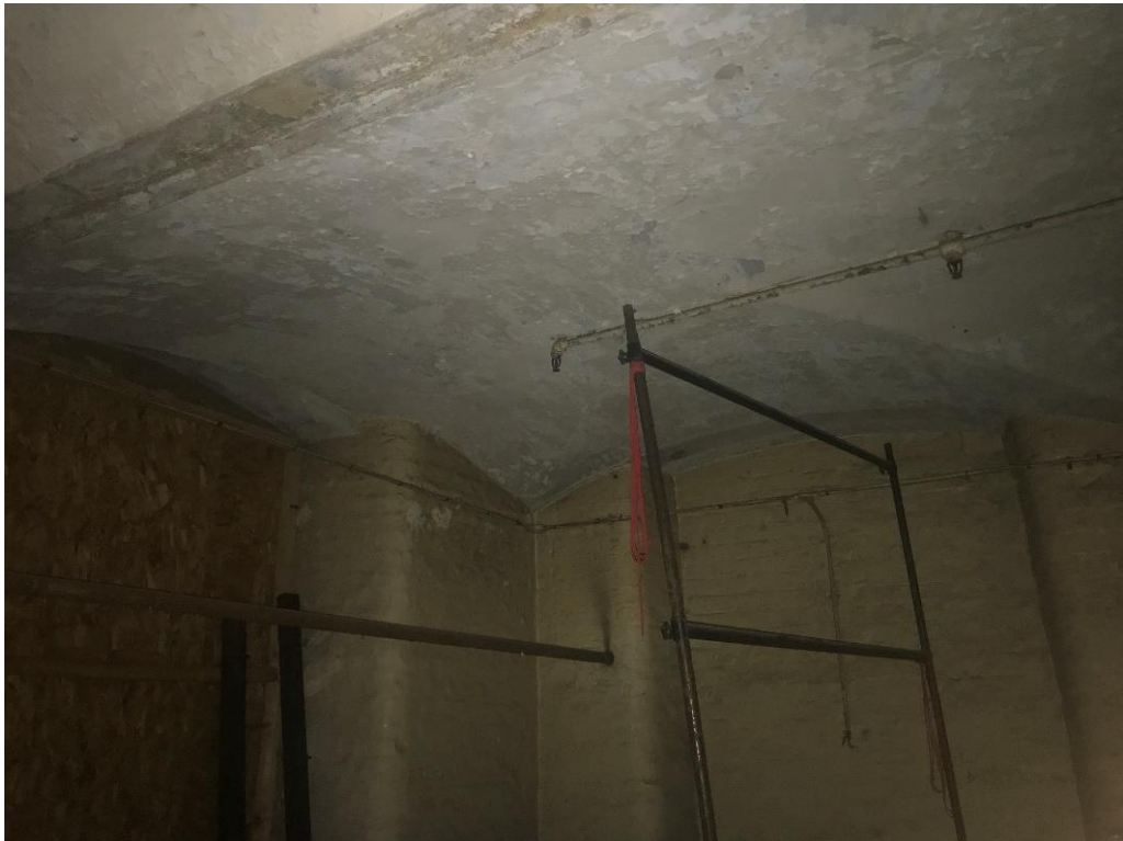
Figure 7: Squinch Corner Slab
