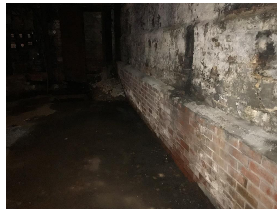
Figure 11: Corbelled Masonry Footing of Main Wing Viewed from within Electrification Tower
