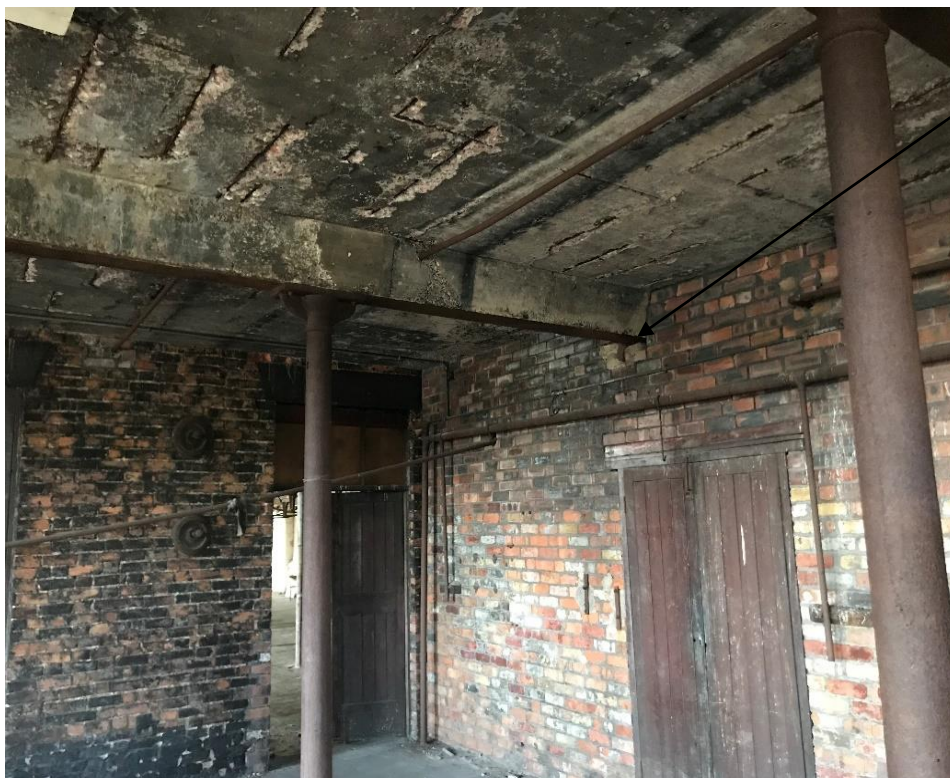
Figure 42: Failed Beam Bearing
