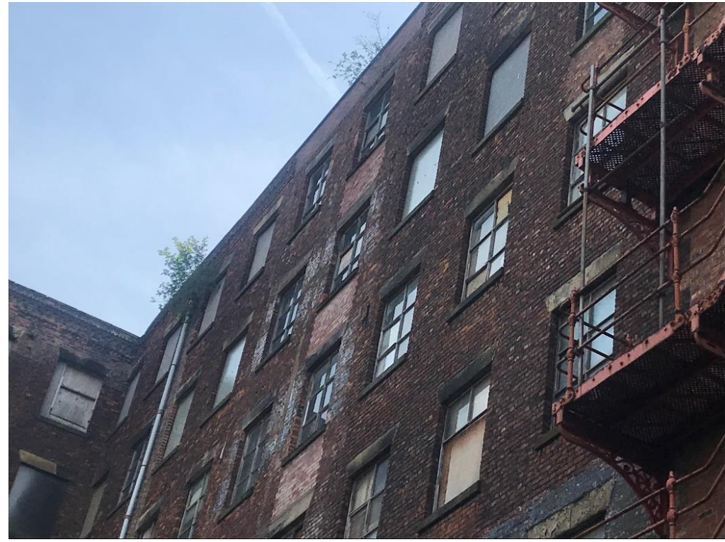
Figure 8: External Solid Masonry Walls
