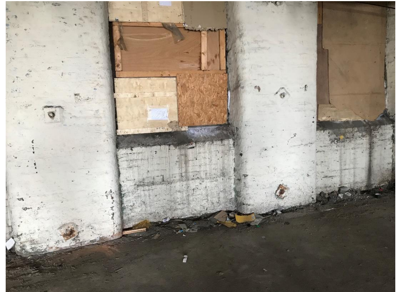
Figure 40: Tie Bars and Plates to Fixed Through Piers
