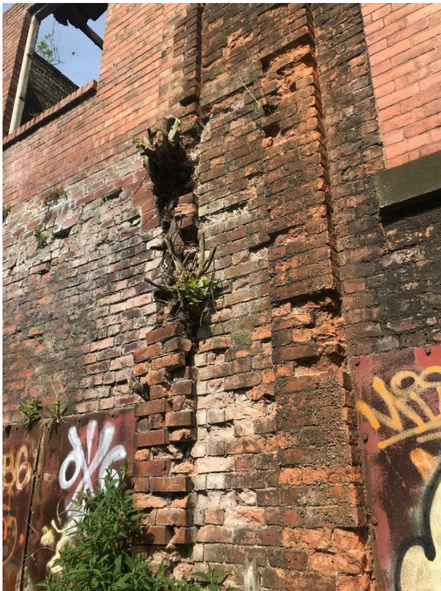
Figure 70: Vegetation Growth Through Pier
