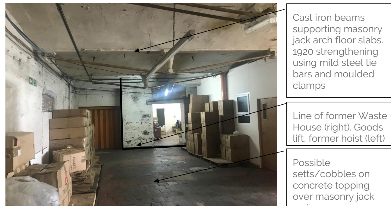
Figure 44: Looking North East into Former Waste House. Goods lift to Left.
