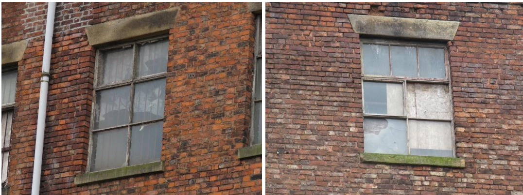
Figure 4 (left): 6 pane window with top two panes hinged at the bottom of the frame to be openable, and Figure 5 (right): 3 over 4 window.
