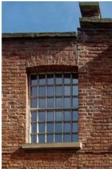
Fig. 1a. Fixed multi-pane window at Murrays Mill, Ancoats.
