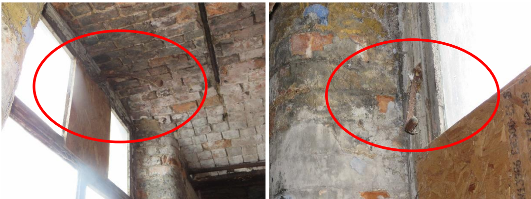
Figures 8 and 9: Internal view showing opening mechanism and window stay of windows with tilting top pane.
