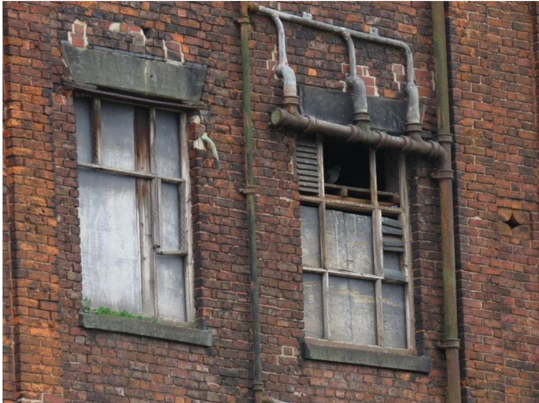
Figure 6: Windows with ventilation louvre panels.
