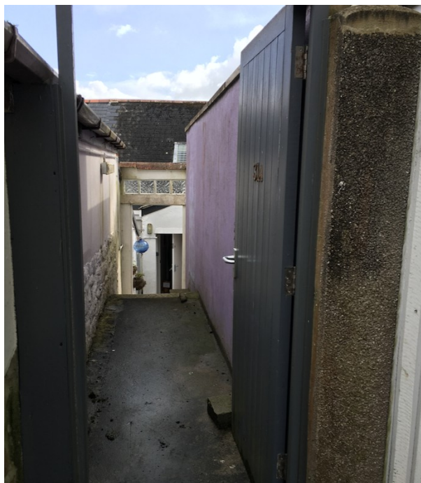
Entrance to the rear of No. 31 from Bread Street
