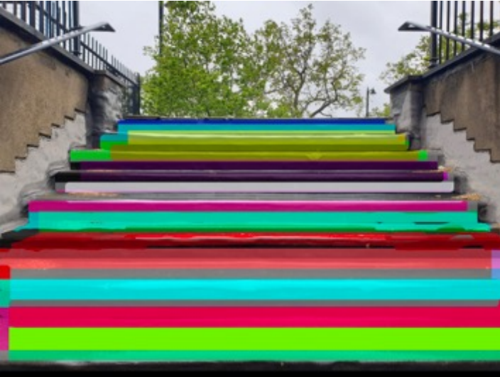
Steps to be coloured tread and upstand using temporary outdoor grade non-slip vinyl
