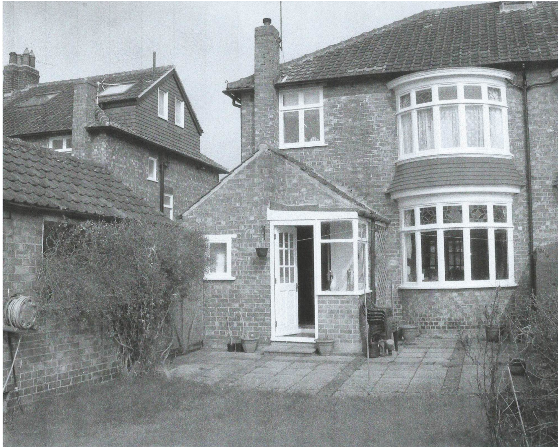
Photograph 1. Rear elevation showing single story outrigger and side elevation of detached garage.
