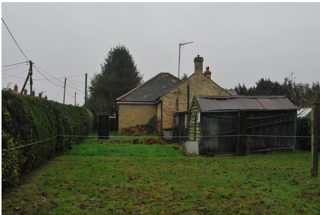
A view of the existing single storey property to be demolished
