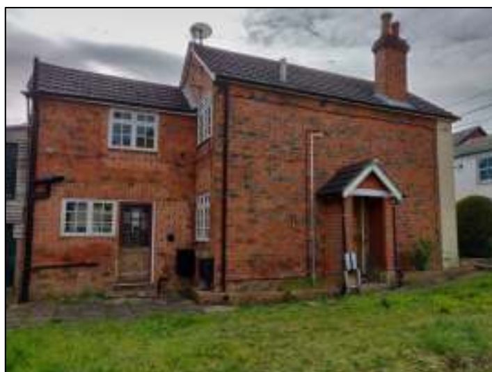
Photo 4.1: Building B1, facing south-west.
