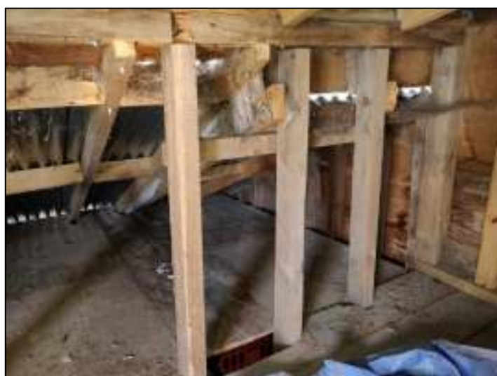
Photo 4.7: Upper roof space of Building B2.
