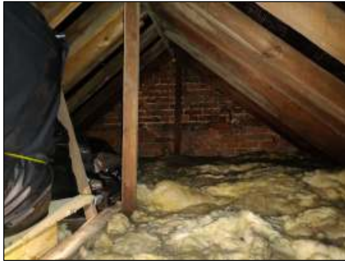
Photo 4.4: Internal loft space in Building B1.
