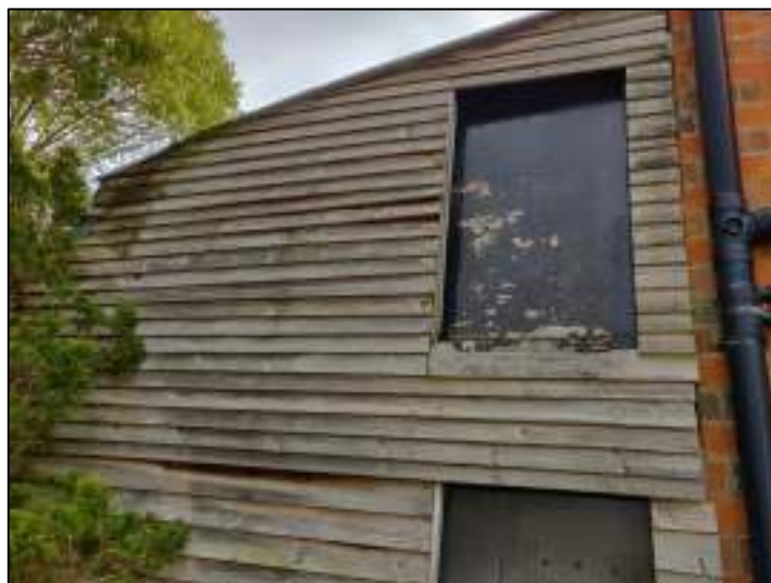
Photo 4.5: Building B2, facing east.
