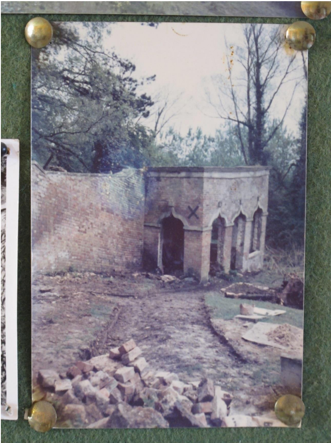
Photo 3: Summer House & wall in 1970s pre-works (©Michael Claydon)
