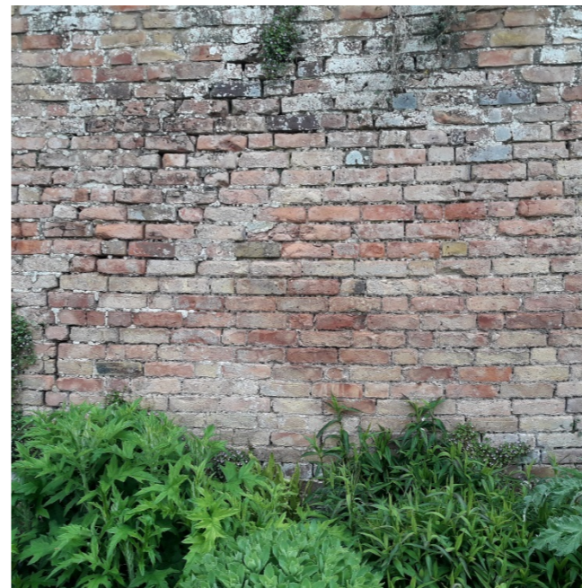
Section H brickwork – no clear bond distinguishable
