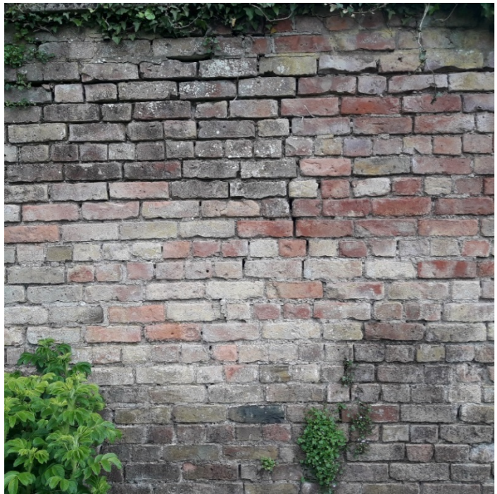
Section F Brickwork more like English Garden Wall Bond
