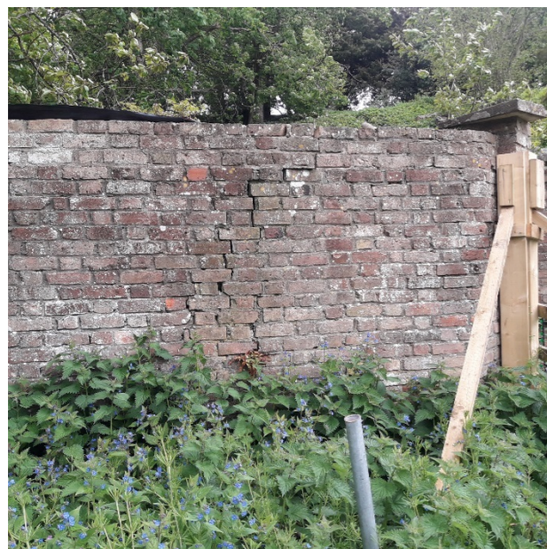
Section E East End Front (1.7m brick repair)
