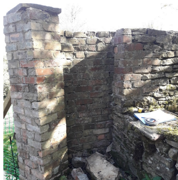
Section E East End Rear (Brick repair)
