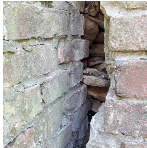
Section E Junction between brick repair and historic wall
