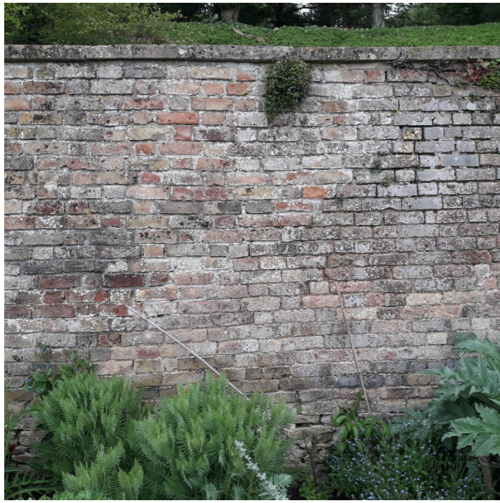
Section J Brickwork primarily Flemish Bond
