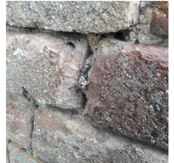
Old nail in Section C brickwork
