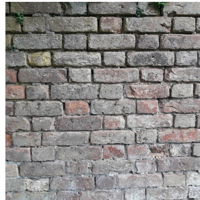
Brickwork to Section C Flemish Bond
