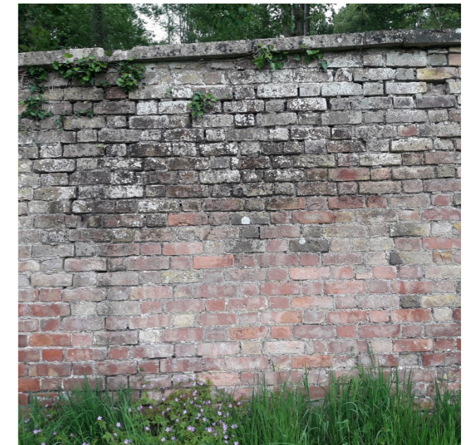
Section A Brickwork – Flemish Bond
