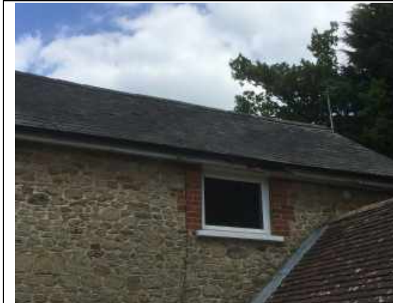
Photo 3 – The slate main roof and tiled extension roof.
