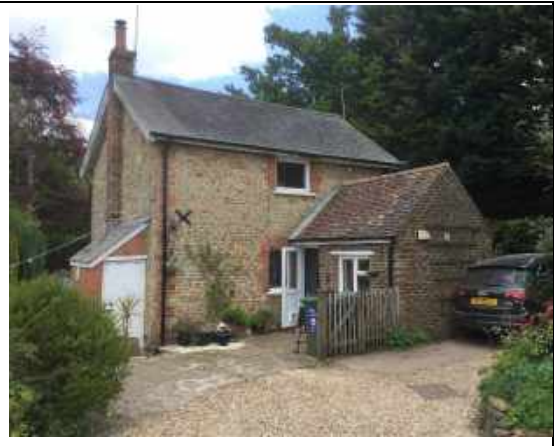
Photo 2 – The west facing elevation and driveway at Wishanger Cottage.
