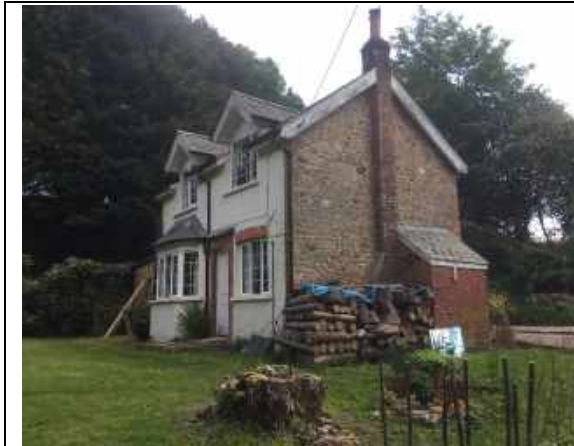
Photo 1 – The north and east facing elevations of Wishanger Cottage.
