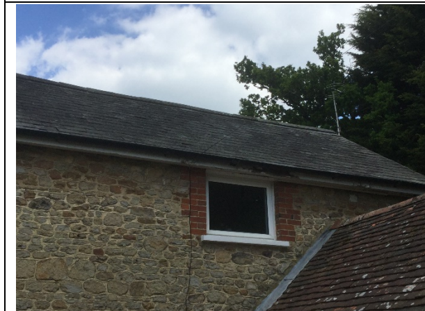
Photo 3 – The slate main roof and tiled extension roof.
