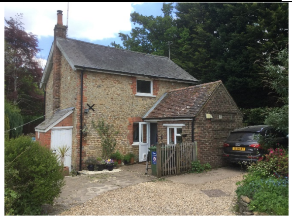
Photo 2 – The west facing elevation and driveway at Wishanger Cottage.
