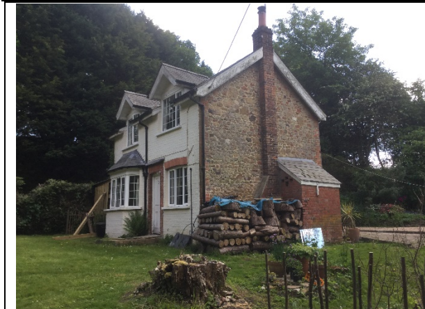
Photo 1 – The north and east facing elevations of Wishanger Cottage.
