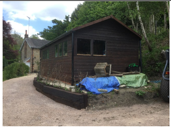
Photo 10 – Timber garage to the west of the site.
