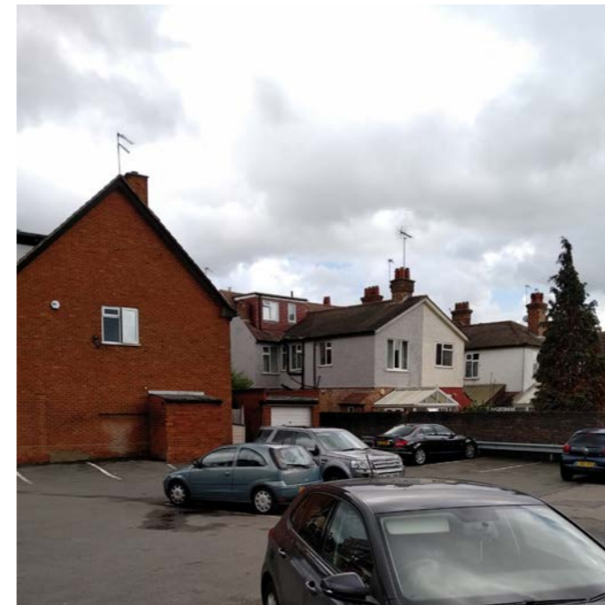
View of west elevation of existing Presbytery and houses
