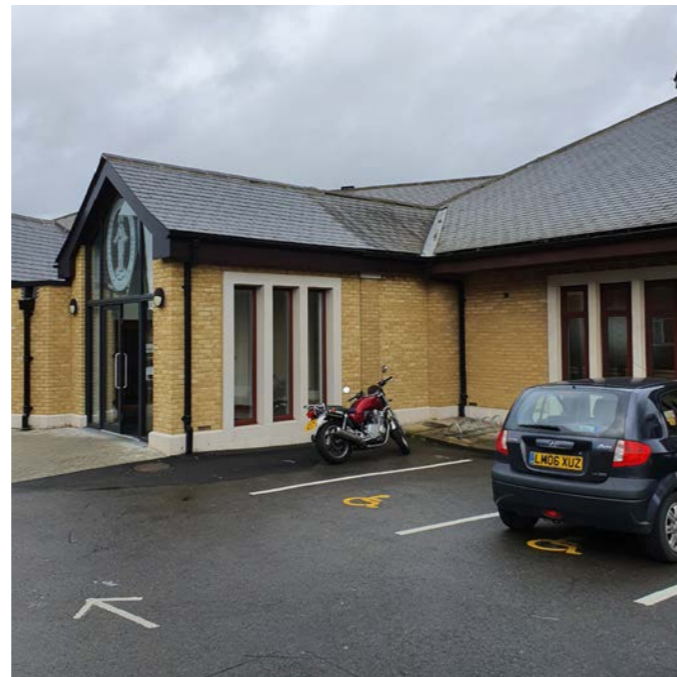
View of recently completed extension
