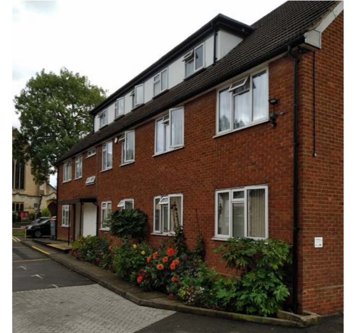
North elevation of existing Presbytery
