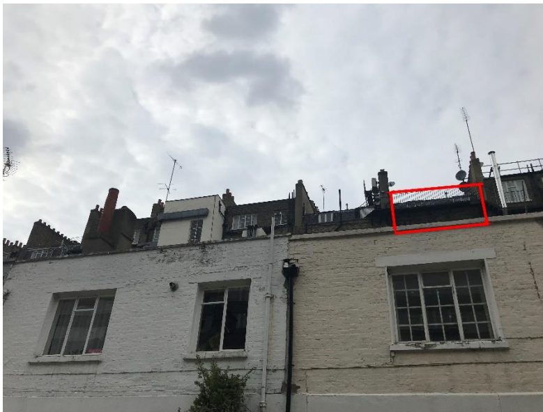
View of the rear elevation of Flat 5, 193 Sussex Gardens from Bathurst Mews
