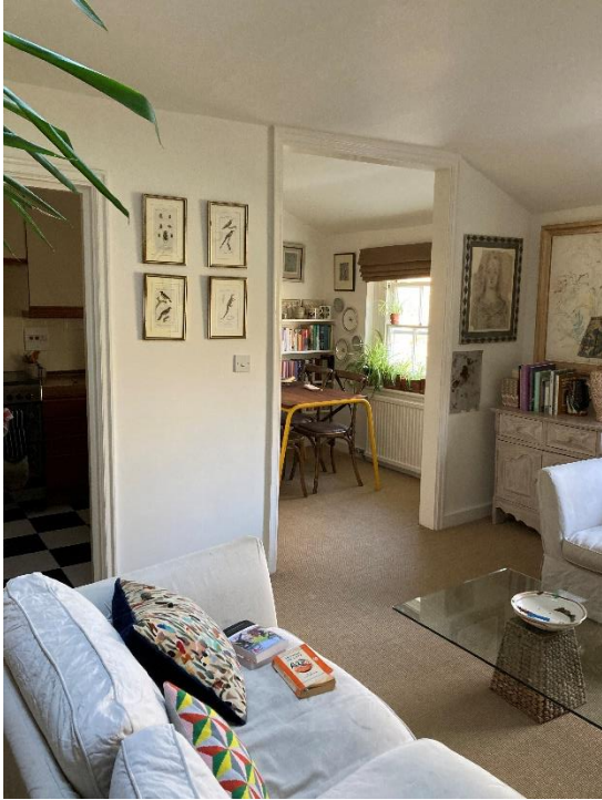
Partition wall and framed openings
