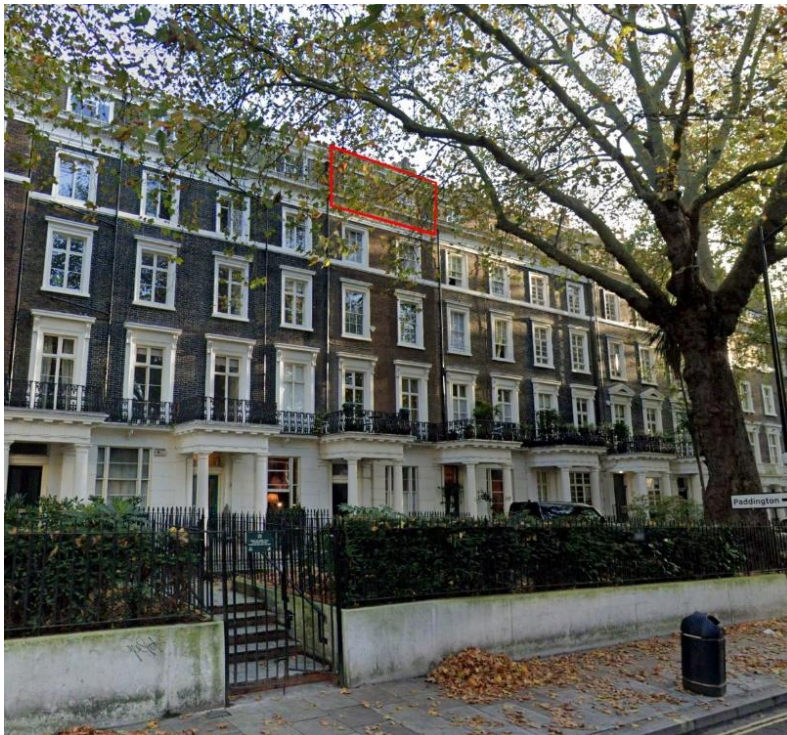
View of the front elevation of Flat 5, 193 Sussex Gardens
