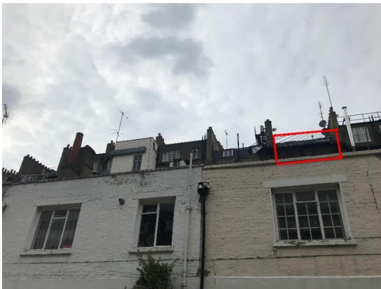
View of the rear elevation of Flat 5, 193 Sussex Gardens from Bathurst Mews
