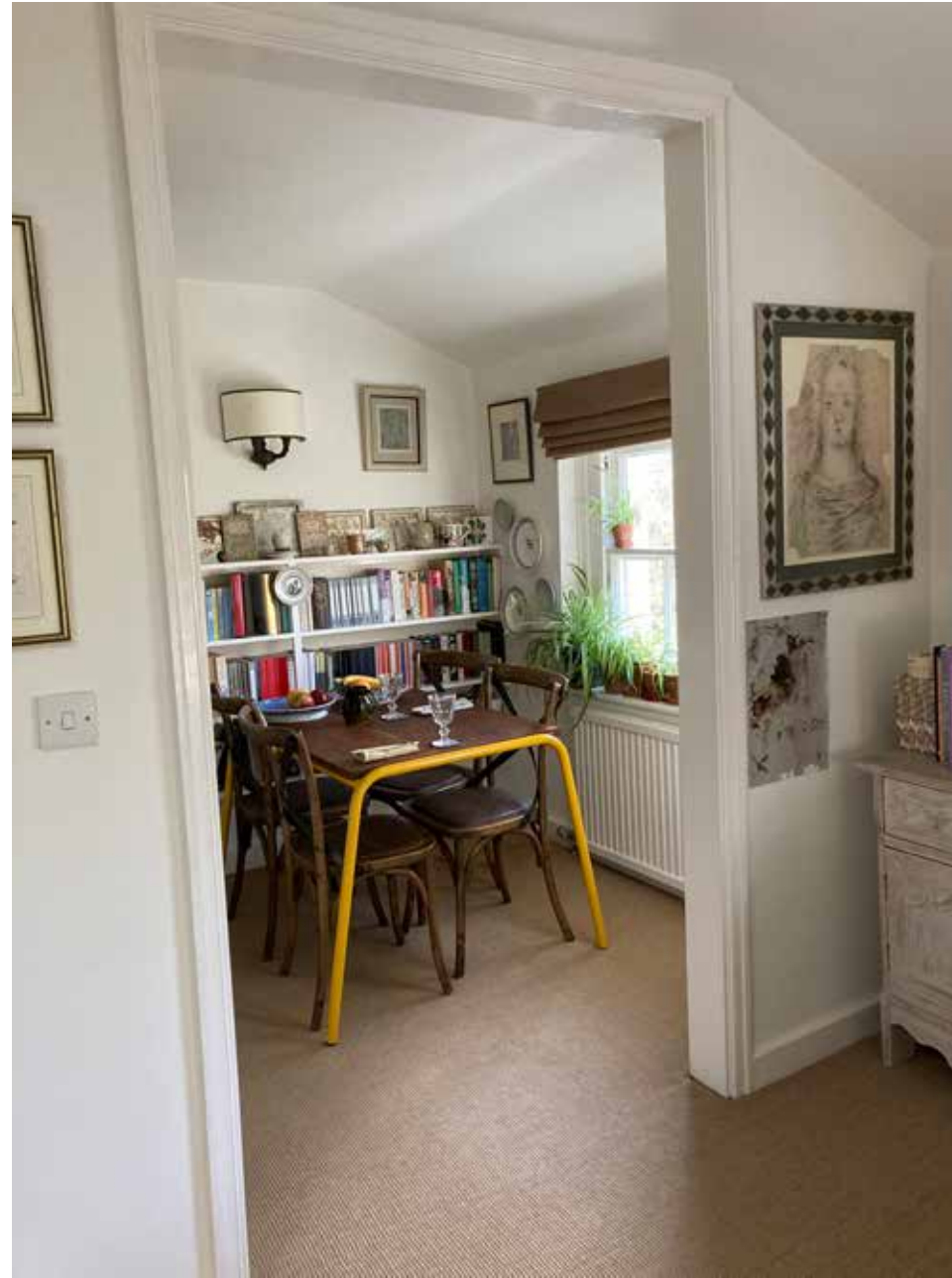
Dining area (Front Elevation) Partition wall to be removed
