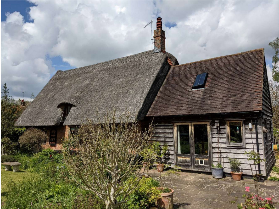
Rear elevation from southeast
