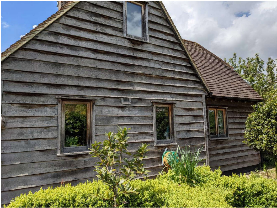
Extension from east
