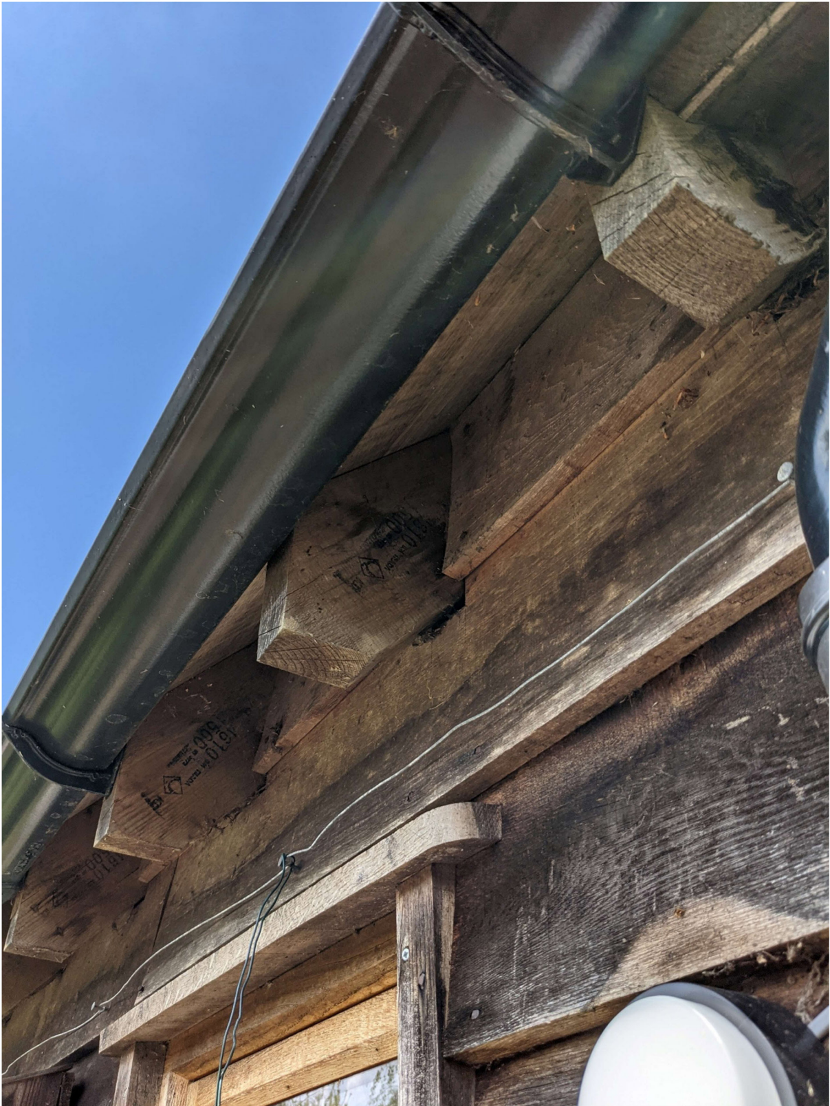
Softwood rafter feet/ends and oak boarding
