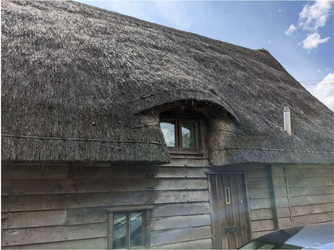
Front elevation and historic front door entrance
