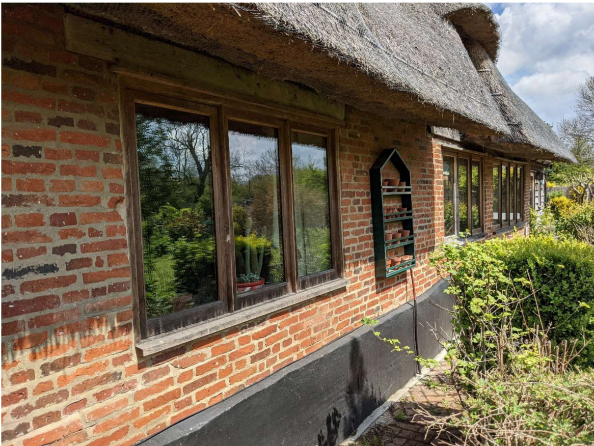
Rear masonry wall of historic dwelling
