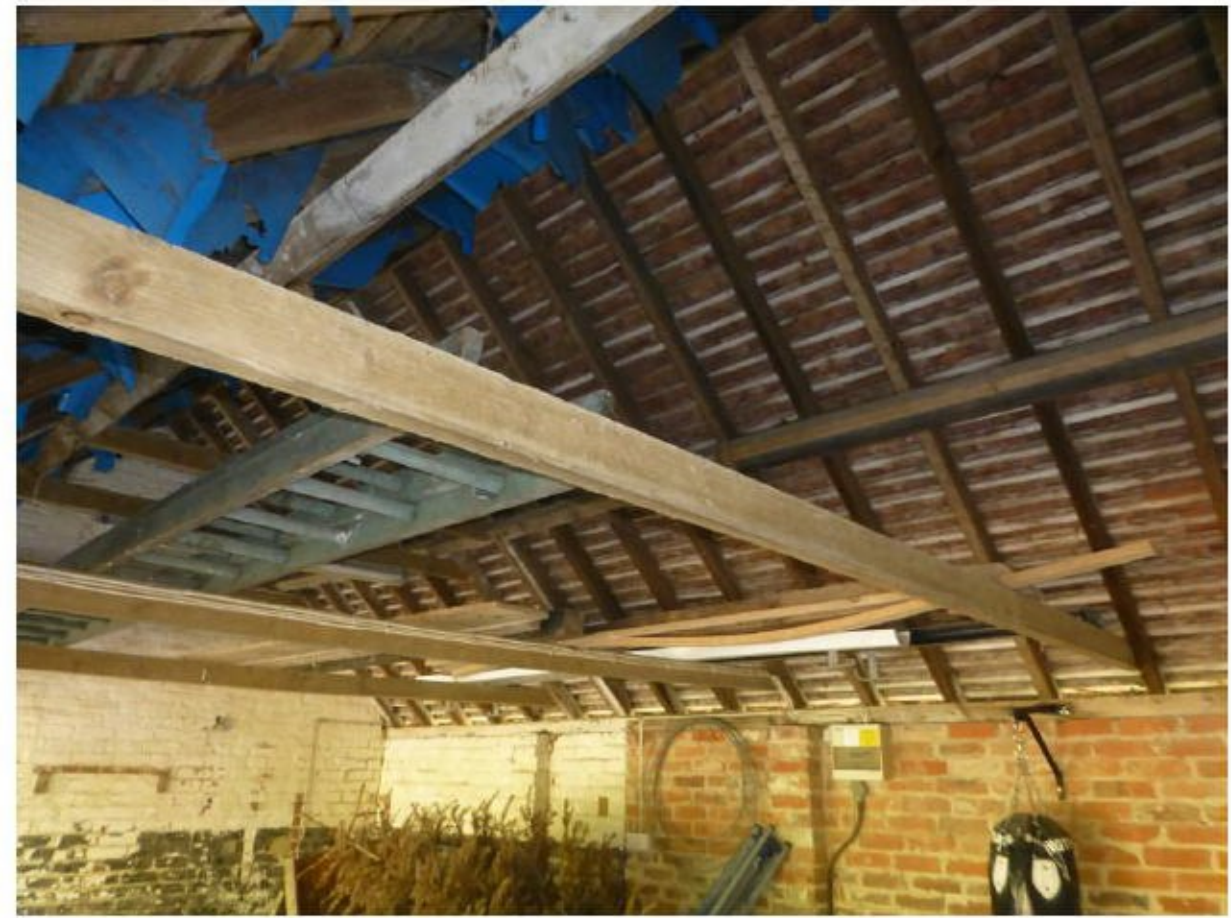
Figure 7. Interior of carport area
