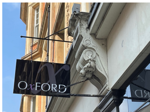
Example of corbel at 12 George Street
