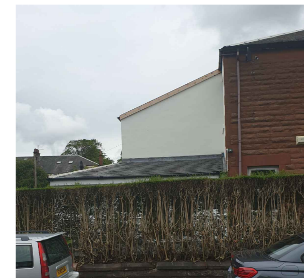
View from side showing existing monopitch roof
