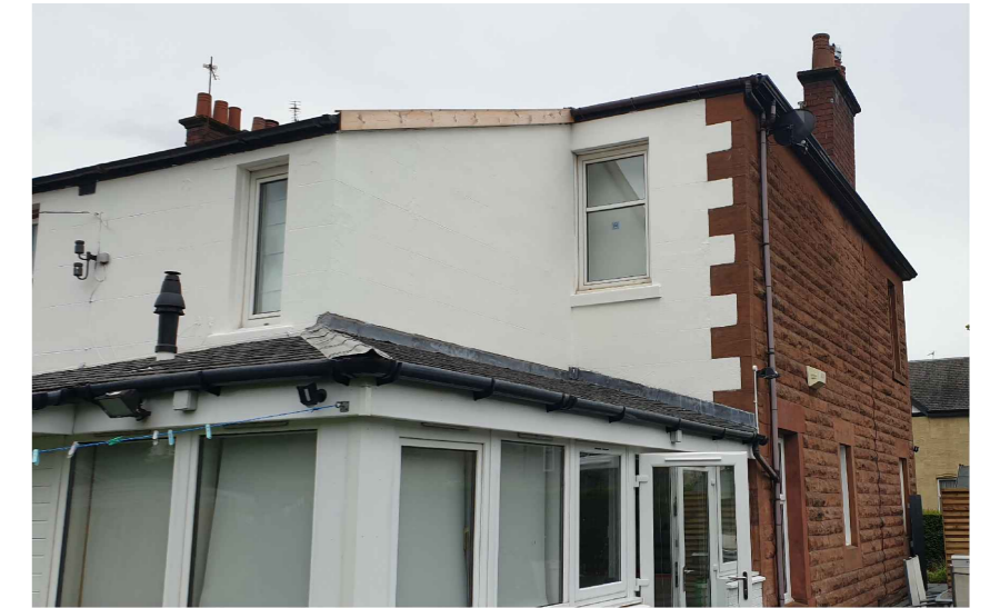
View from rear showing existing monopitch roof
