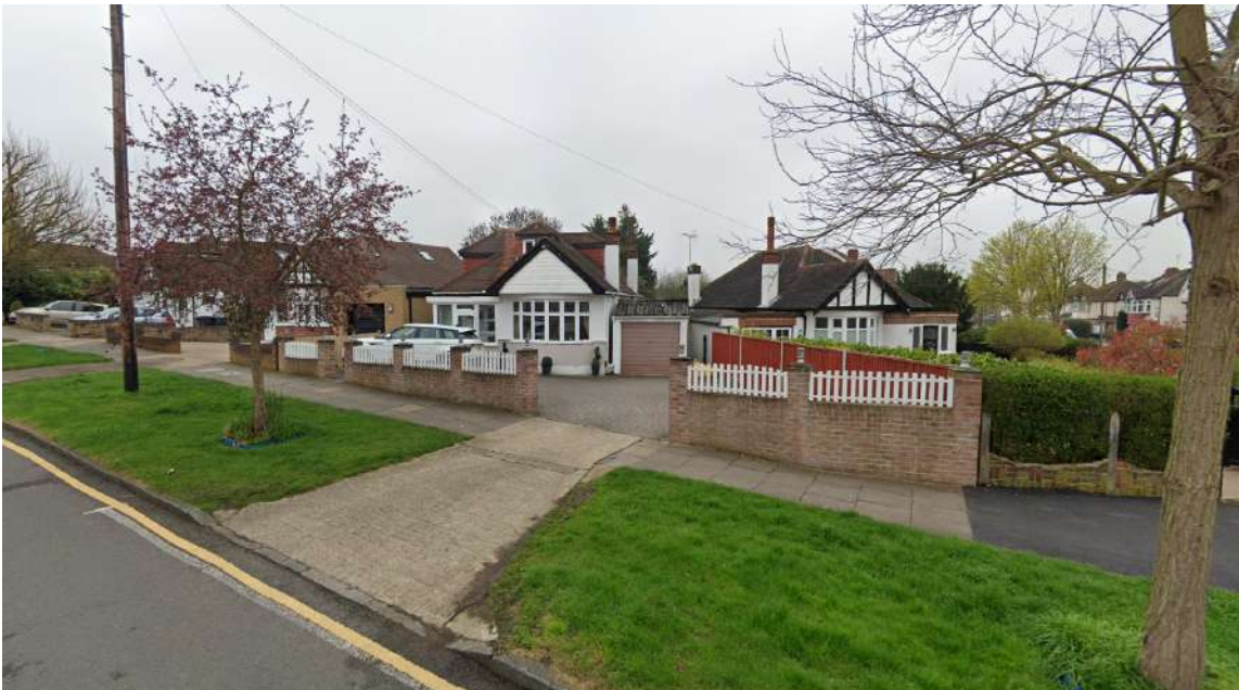
Image 02 - Existing front street elevation
