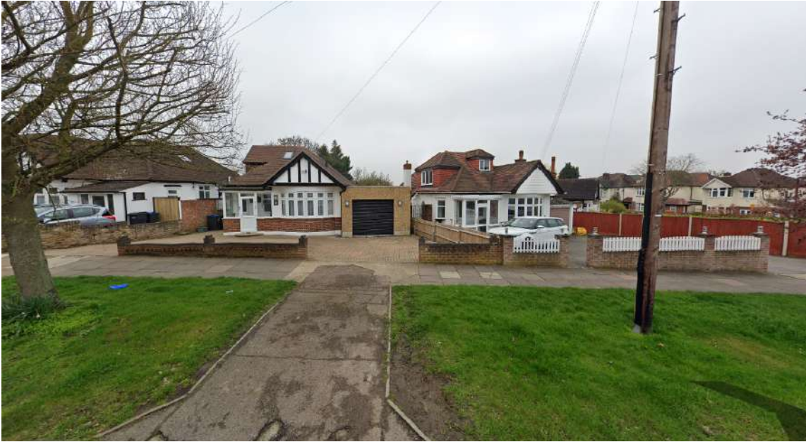
Image 01 - Existing front street elevation
