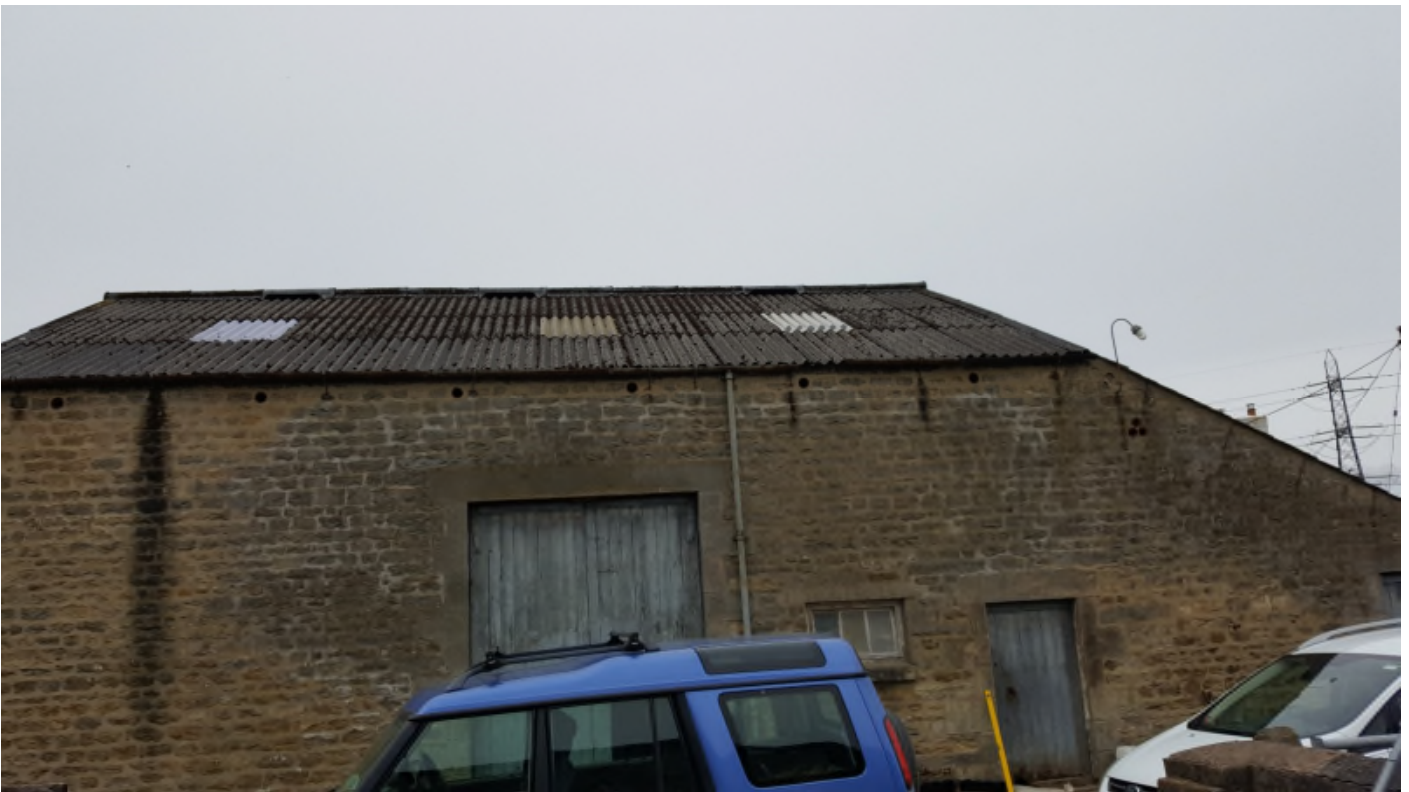
Roof profile from Wall 1
