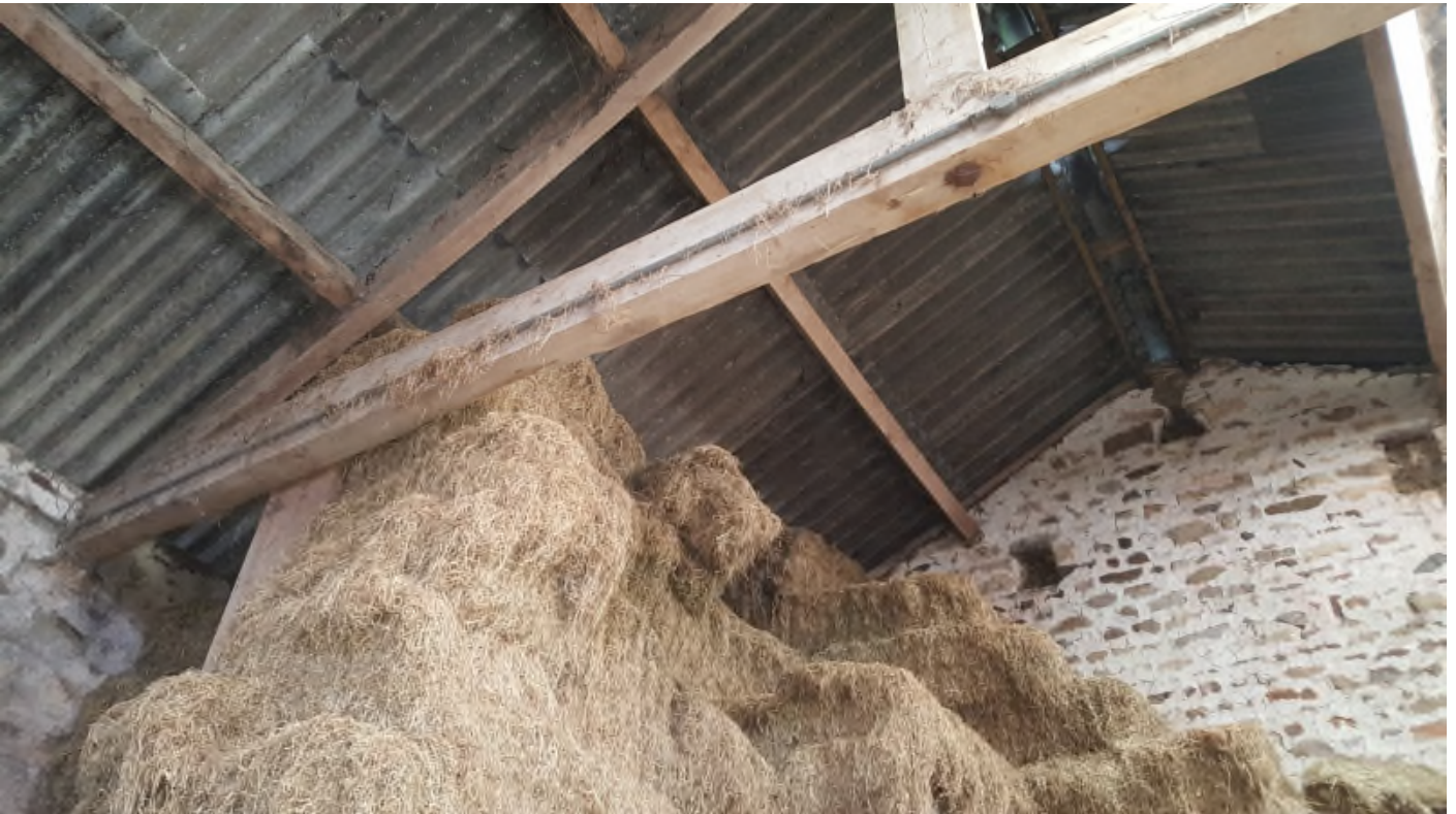
Internal – Hay loft above work room – two storey section
