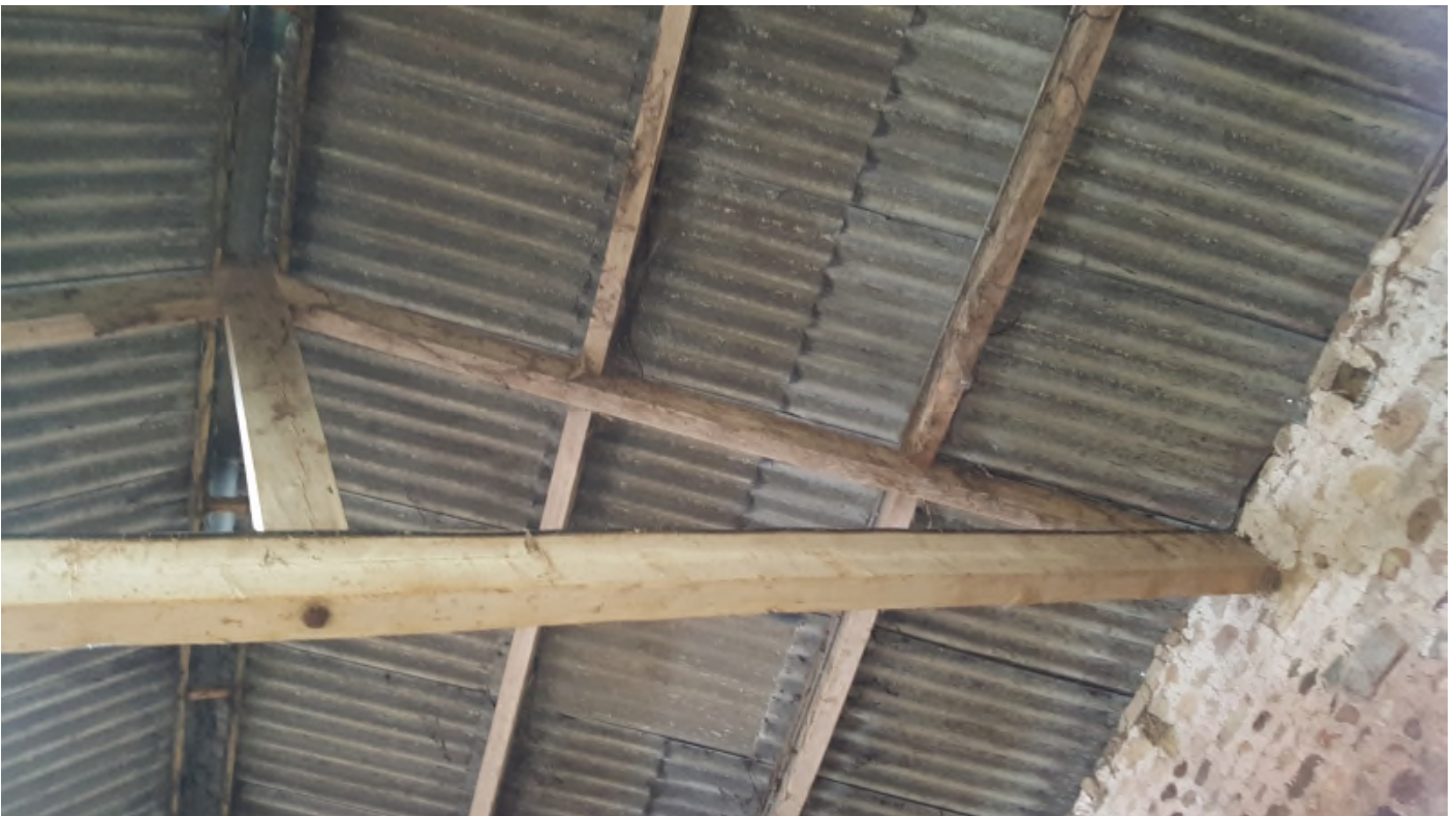
Internal – two storey section – showing king post truss and sheeted roof
