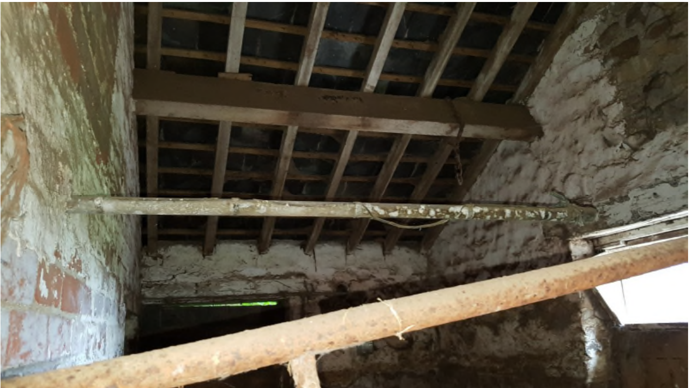
Internal – Single storey section – South elevation/Wall 2 Traditional purlin and rafter construction clad with slate
