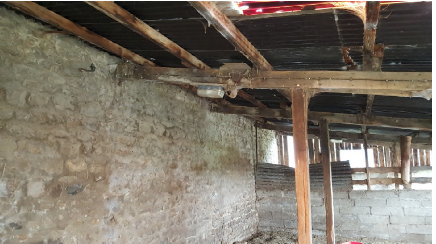
View of Wall 4 from within outbuildings
