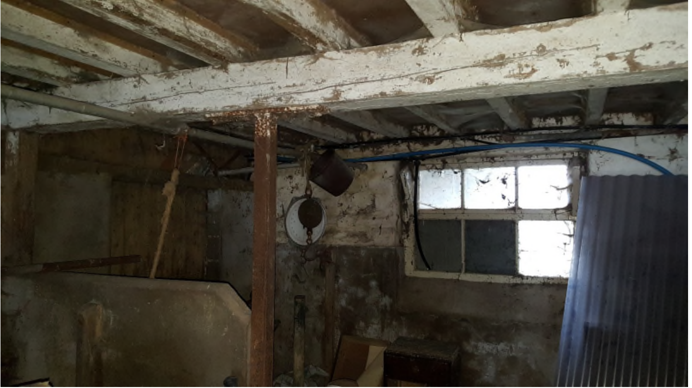
Internal – Work room (hay loft above)
