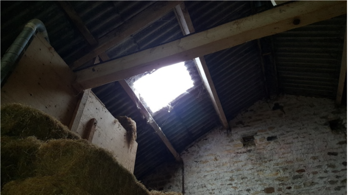
Internal – two storey section
