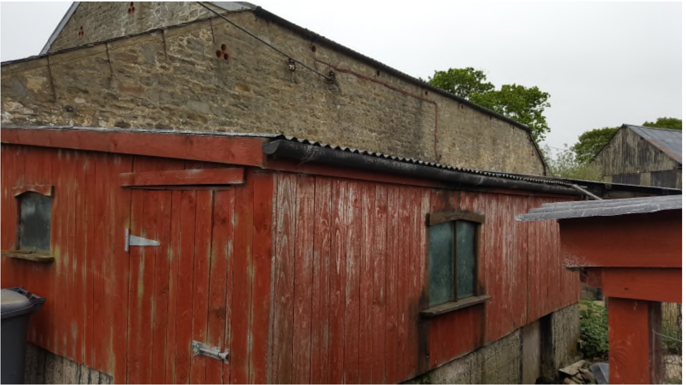
Wall 4 – Block/timber clad outbuilding omitted from this report
