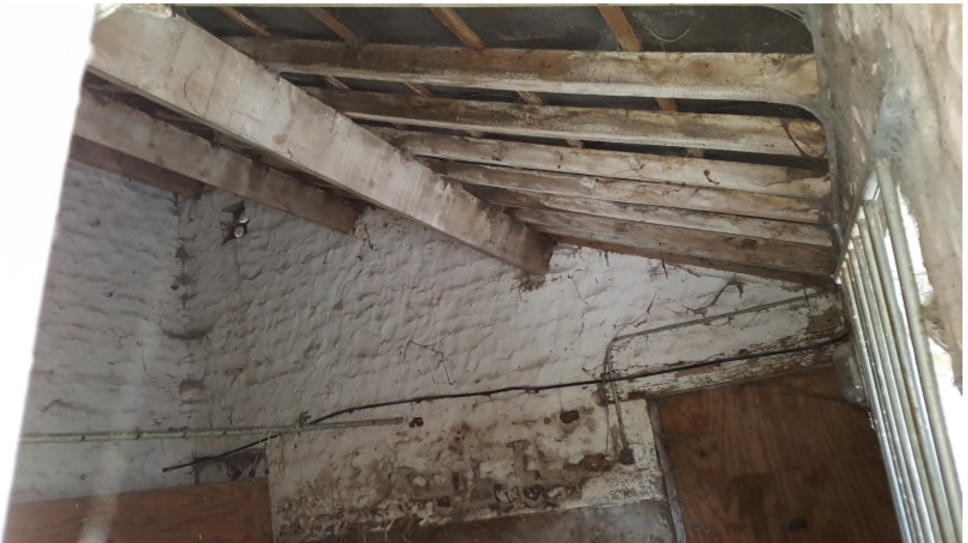
Internal – Single storey section – North elevation/Wall 3
