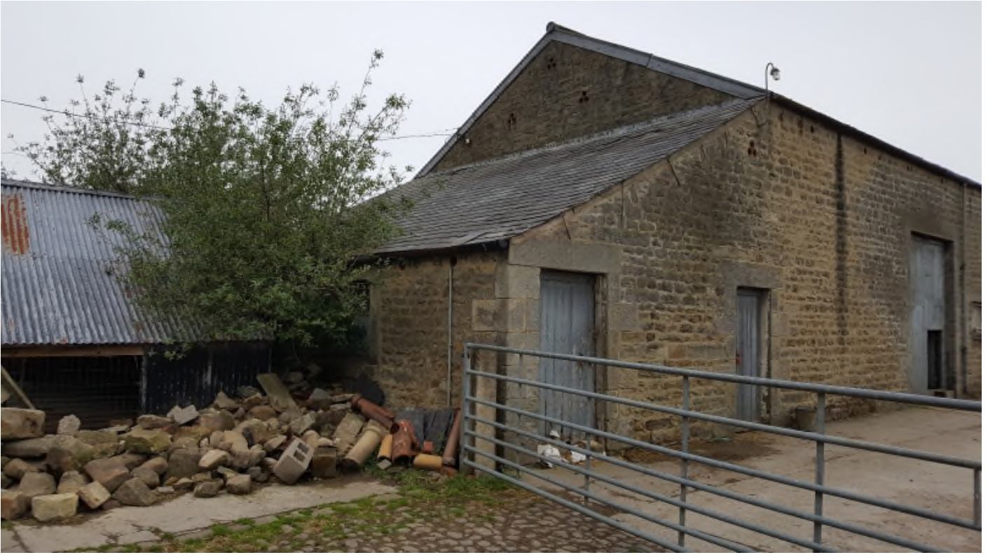
Single storey section to South
