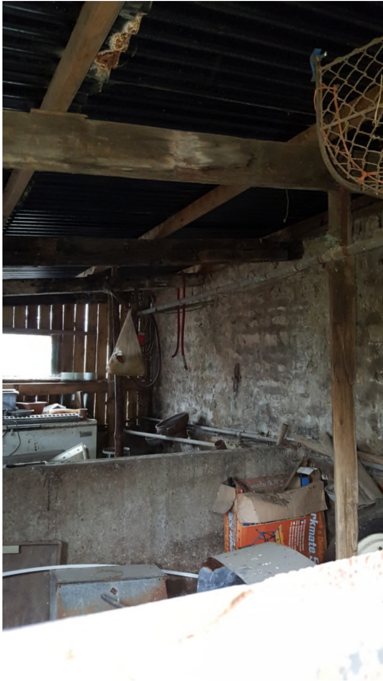
View of Wall 4 from within outbuildings
