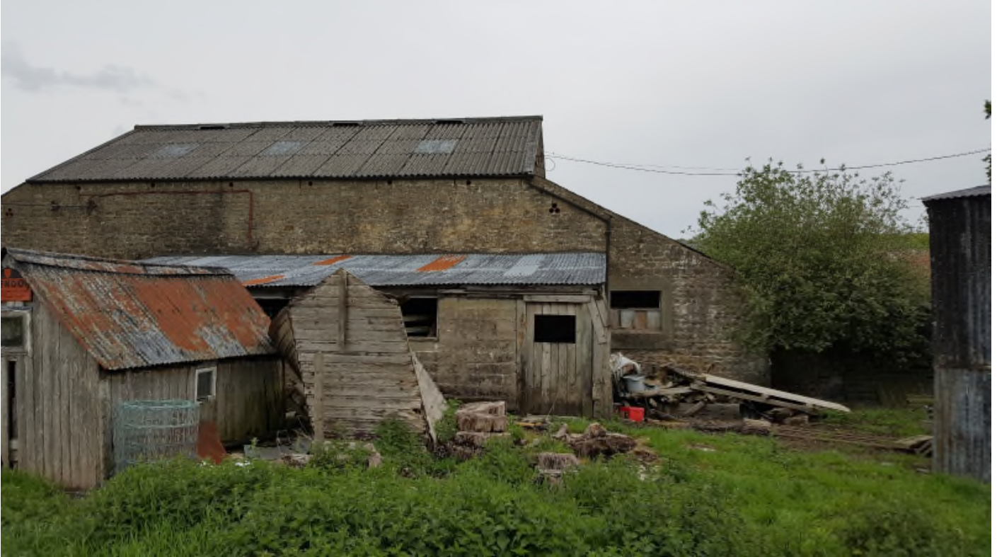
Roof profile from Wall 4
