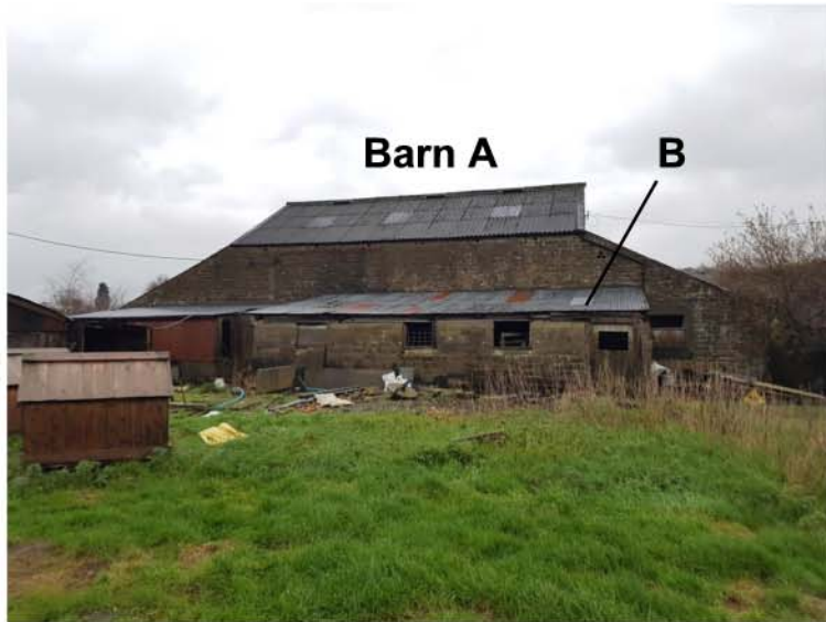
view of site looking northeast
