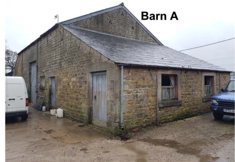
view of site looking south
