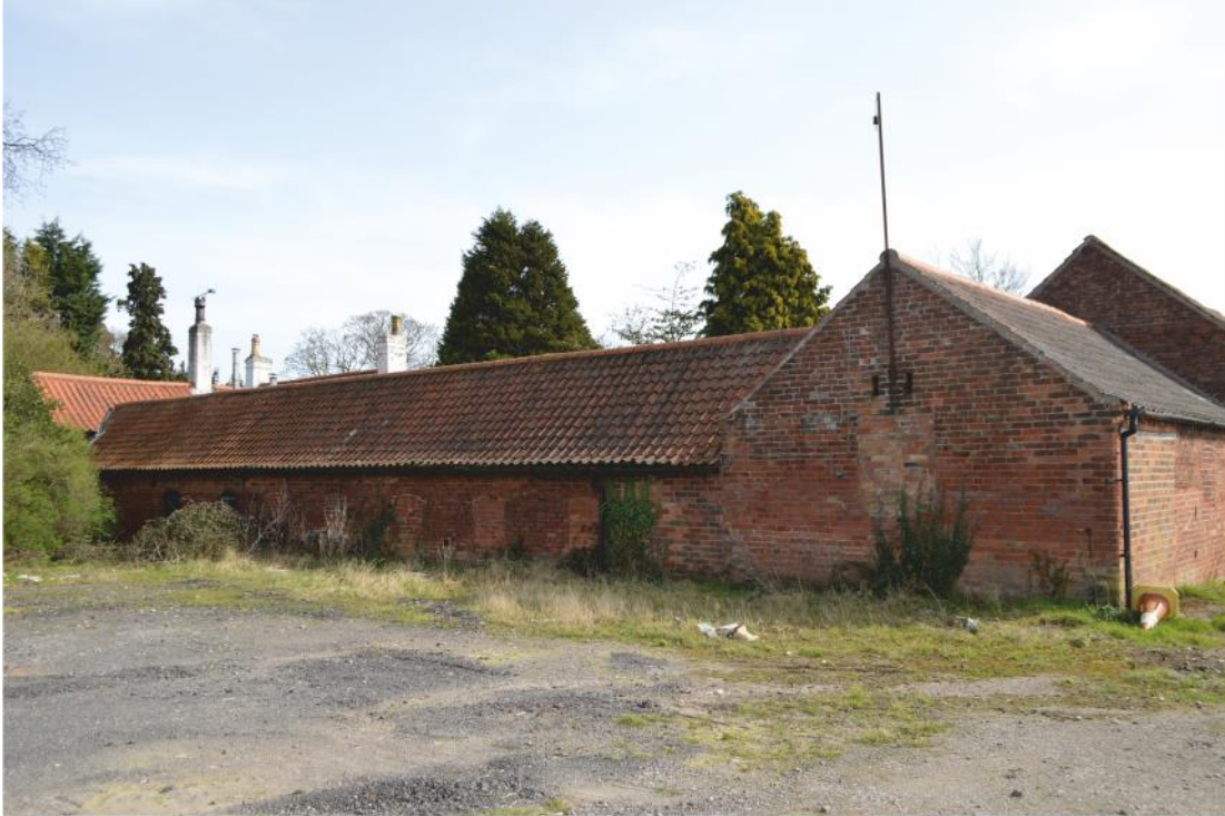
PI.15 Cowshed overlooking the development site, showing blocked openings
