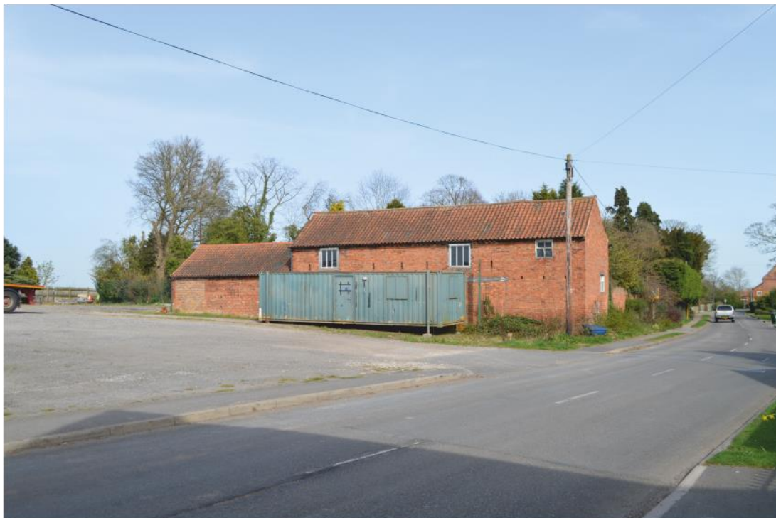
Pl. 14 Barn and cowshed (left) west of Priory Farmhouse overlooking the development site
