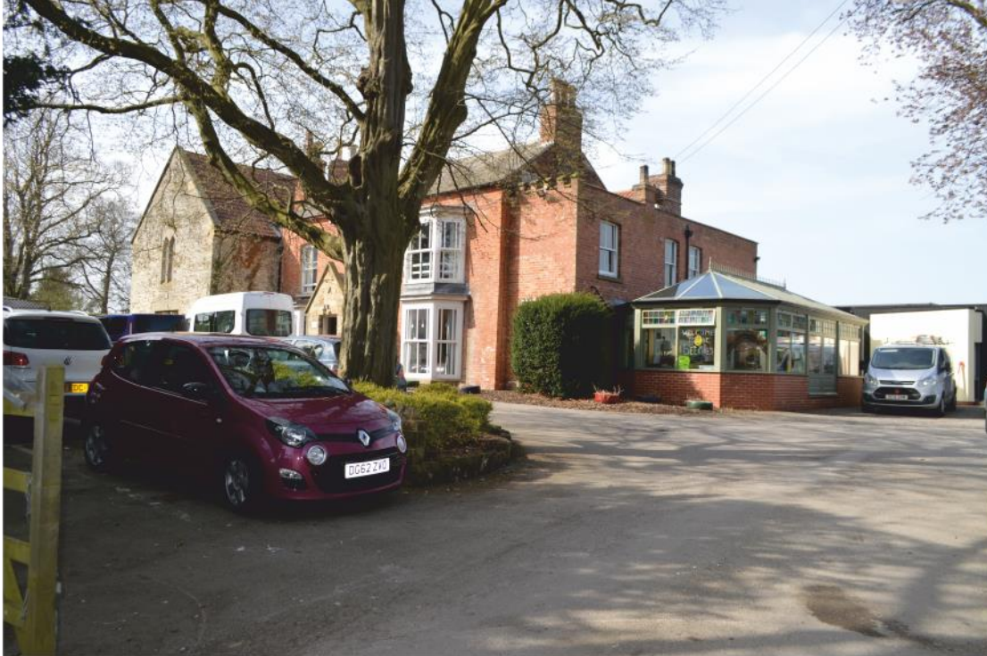
Pl. 7 The Priory, looking north-west from Retford Road entrance
