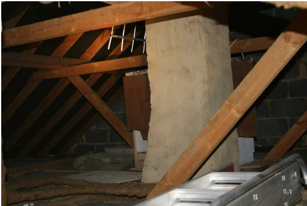
Figure 4: View across Roof Void
