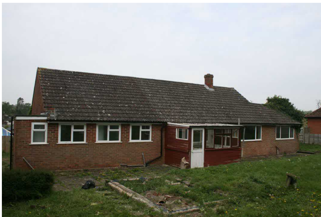
Figure 1: View of east elevation of bungalow (rear garden)
