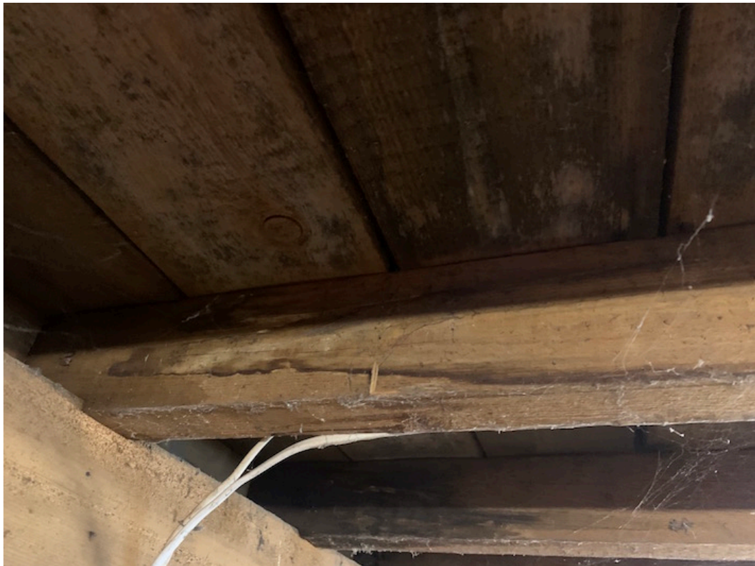
evidence of historic water ingress (above + below) as well as signs of mould growth to roofing timbers
