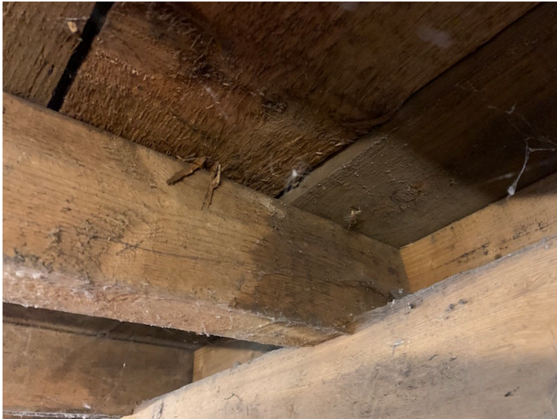
evidence of recent/current water ingress (above) and more historic water ingress (below)
