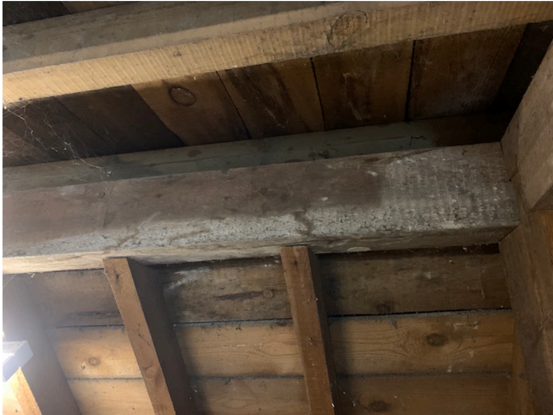
evidence of historic water ingress (above + below) as well as signs of mould growth to roofing timbers
