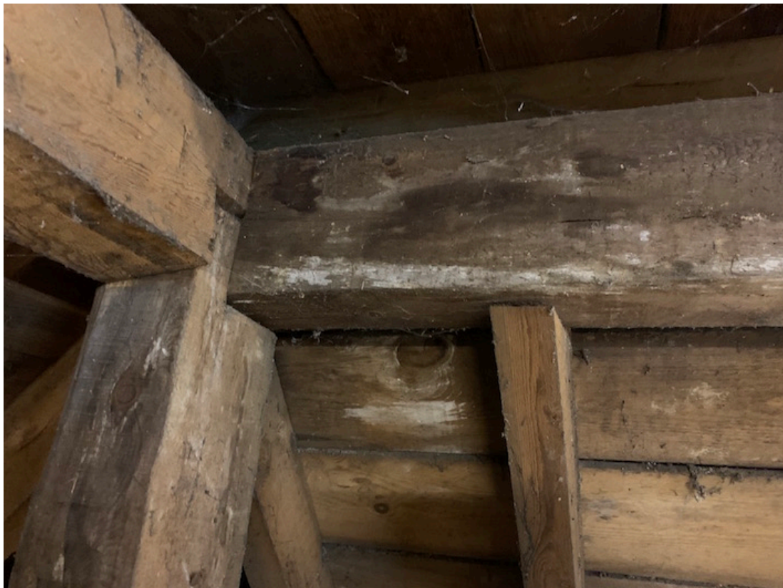
evidence of recent/current water ingress (above) and more historic water ingress (below)
