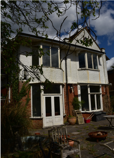
View of Hill House from the South
