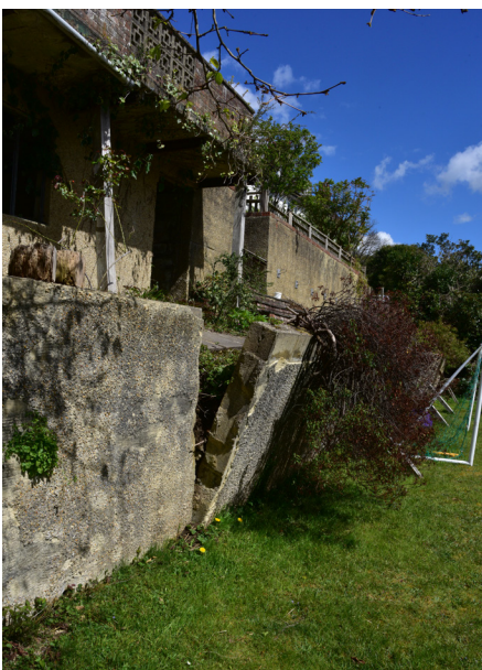
View of the middle retaining wall
