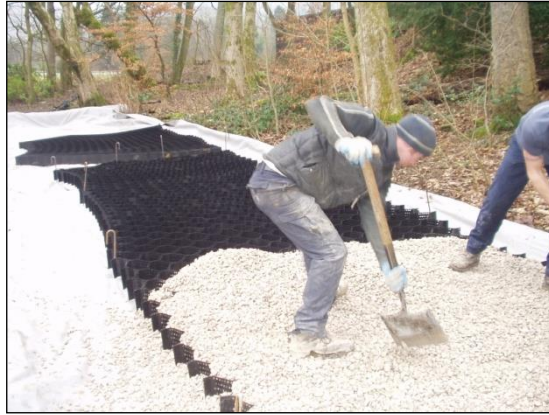
Photo 3- expanding and filling the Cellweb system
