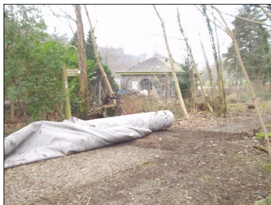
Photo 2- laying of Fibretex material onto existing subgrade
