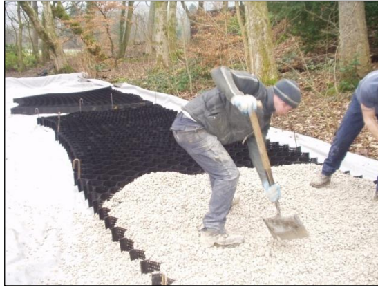
Photo 3- expanding and filling the Cellweb system
