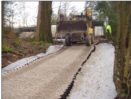
Photo 4- once filled the system can support plant to carry aggregate to the fill area
