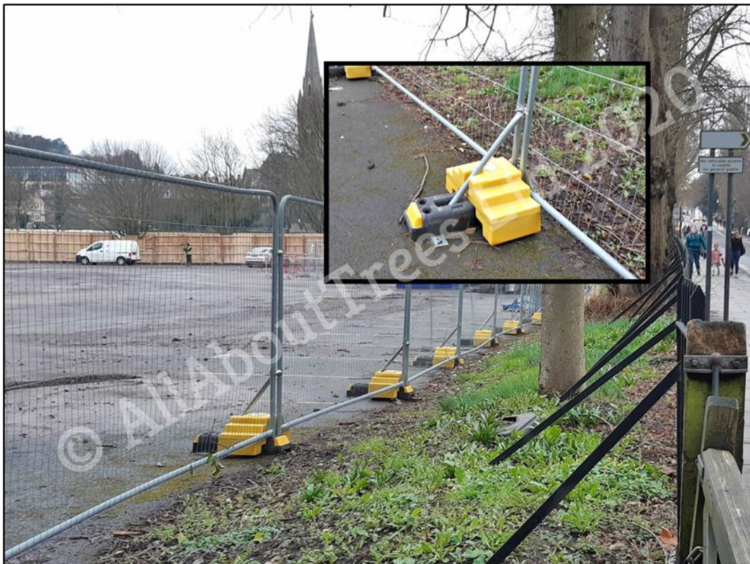
Figure 2 – An example of a barrier erected on a site
