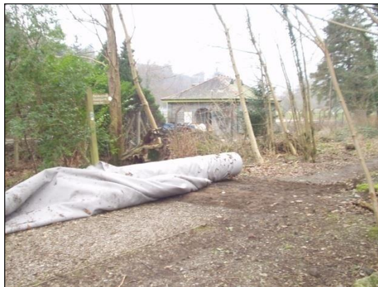
Photo 2- laying of Fibretex material onto existing subgrade
