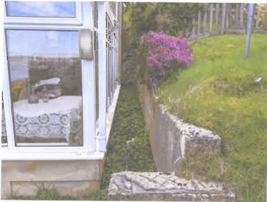
South side of house
