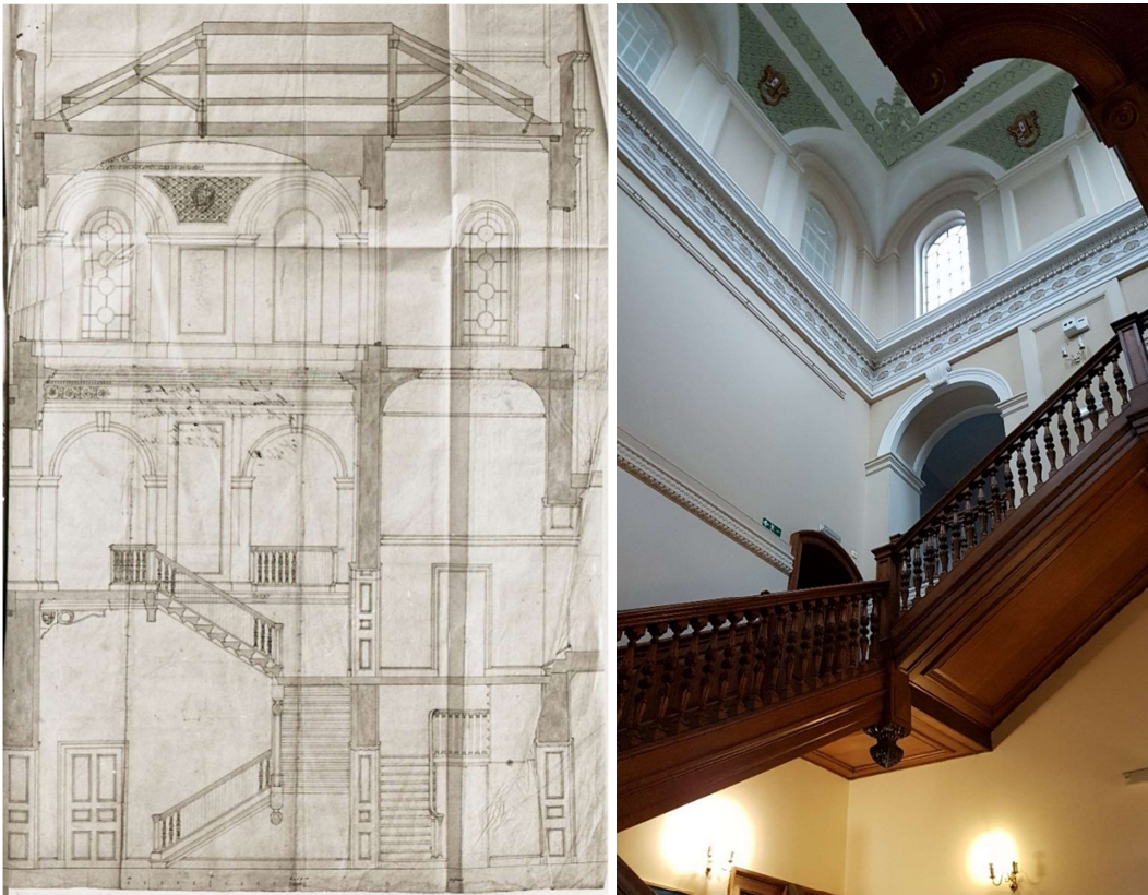
Figure 1: Grand timber staircase and cantilevering balcony within decorated lantern.
