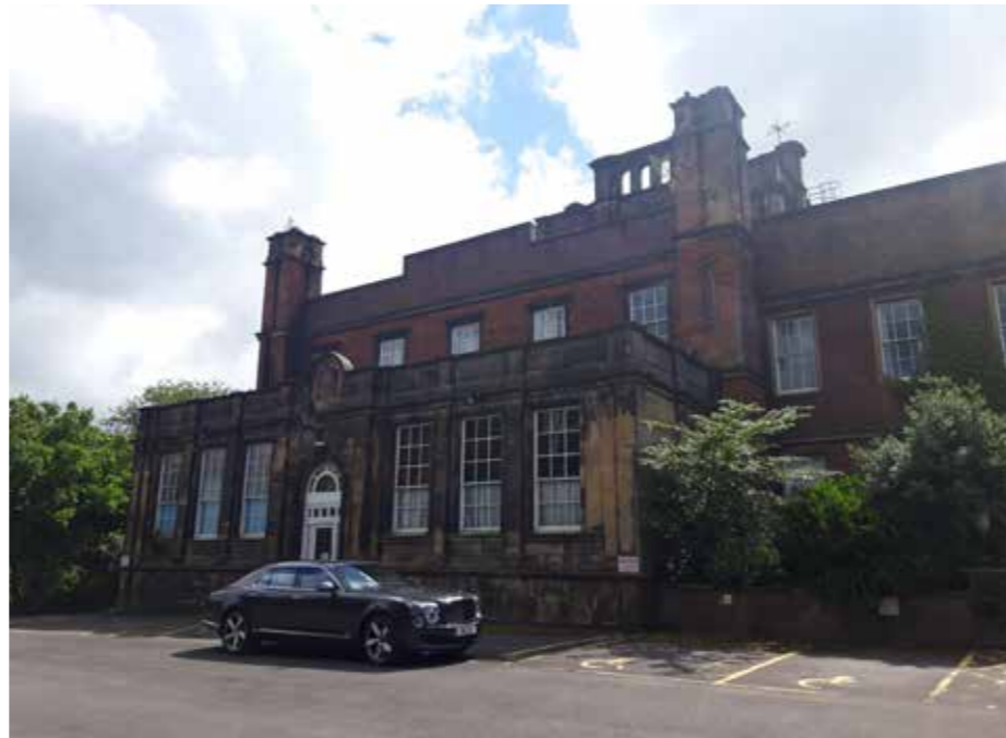
View of the north front showing the later porch extensions added to Lewis Wyatt's entrance front.
