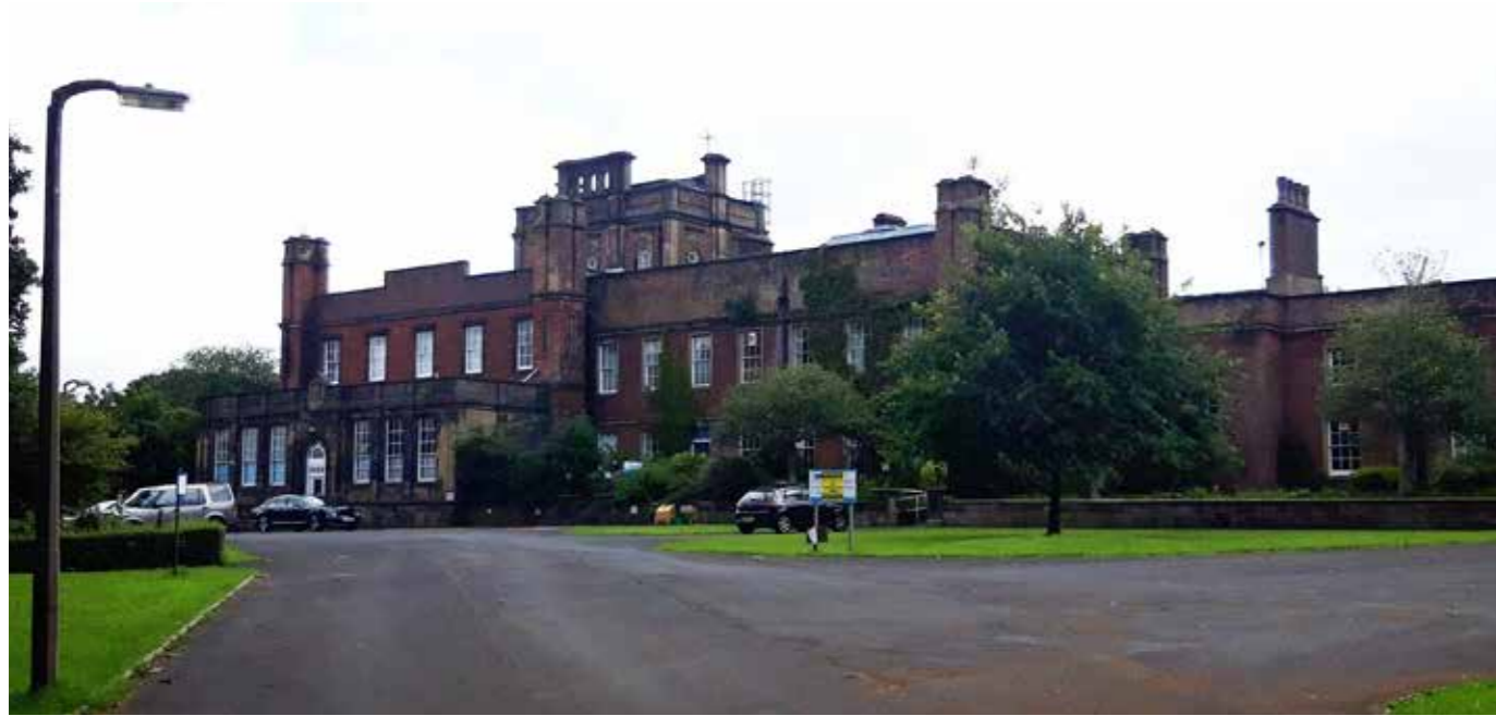
Above: View of Cuerden Hall from the entrance drive as existing.
