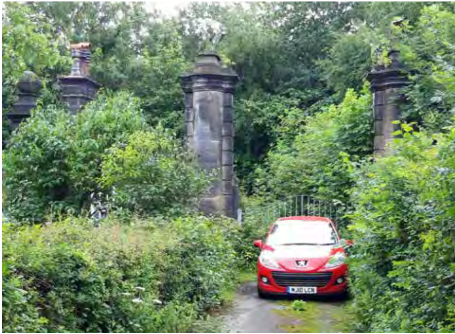
View of Stag Lodge, Wigan Road, the former principal carriage drive entrance to Cuerden Hall.
