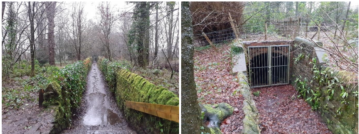
Figure 2: Pathway looking north (left) and south entrance of tunnel (right).
