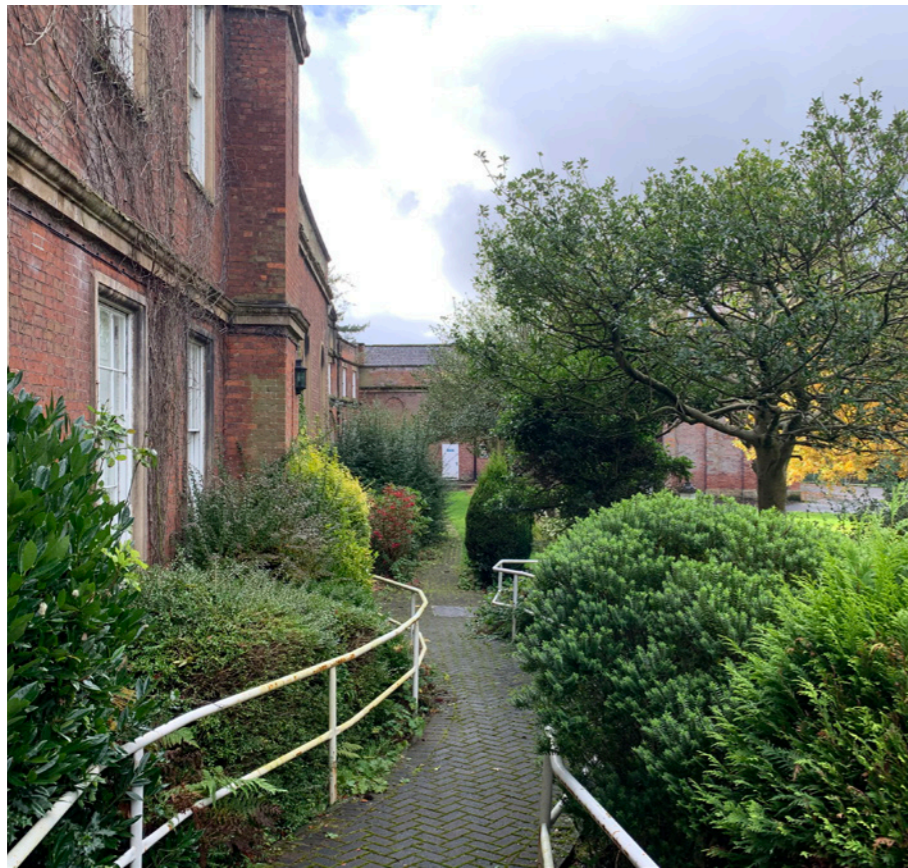
Curved ramp to main entrance
