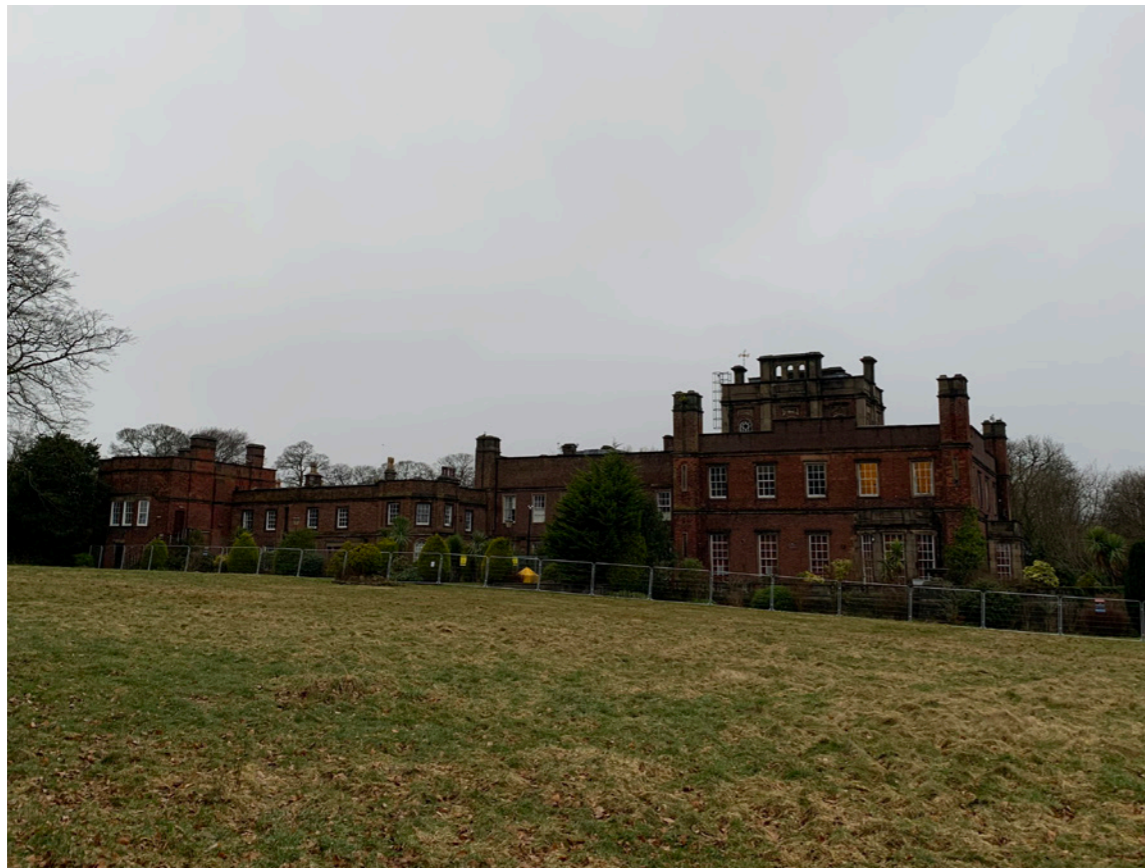
Southern facade of Cuerden Hall and sloping southern lawn
