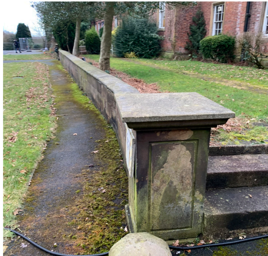
Existing walls along northern elevation
