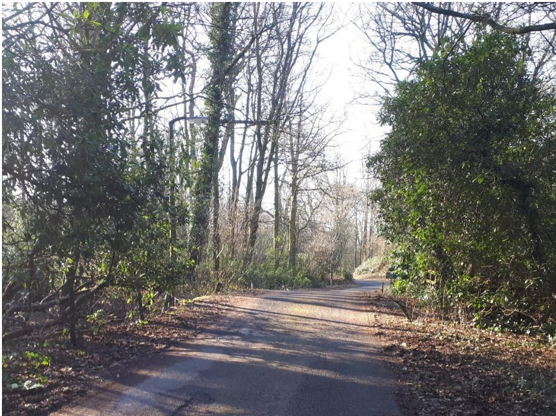
Figure 7: View of the hump in the road above tunnel looking west.
