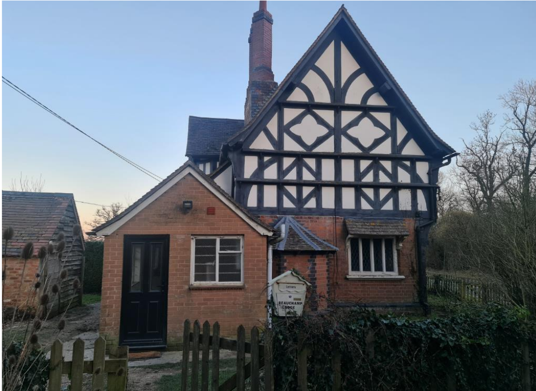
Figure 2: Front (west) elevation of Beauchamp Lodge
