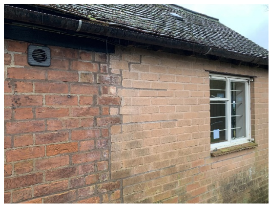
Figure 2 Junction of extension
