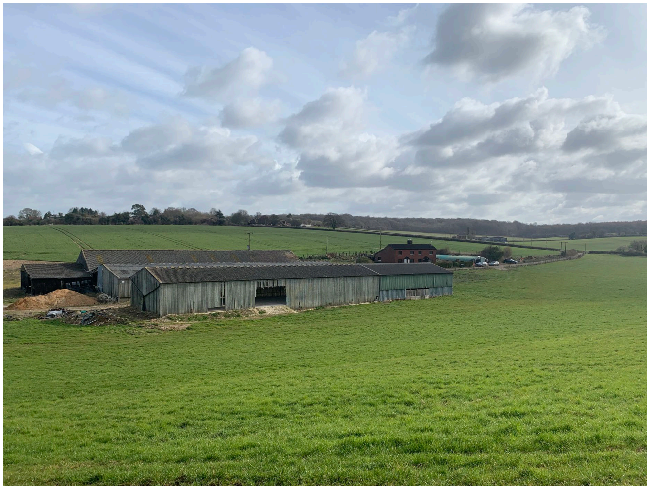
FIG 01 - EXISTING SITE PHOTOGRAPHS
