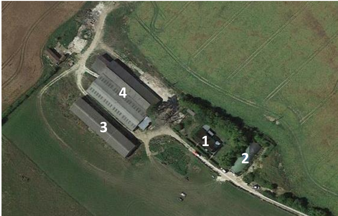
Figure 3: Existing buildings on site
