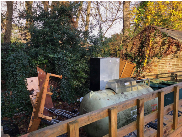
Decommissioned and redundant LPG storage tank to be removed
