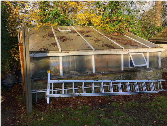
Existing timber and brick built glazed outhouse structure to be demolished
