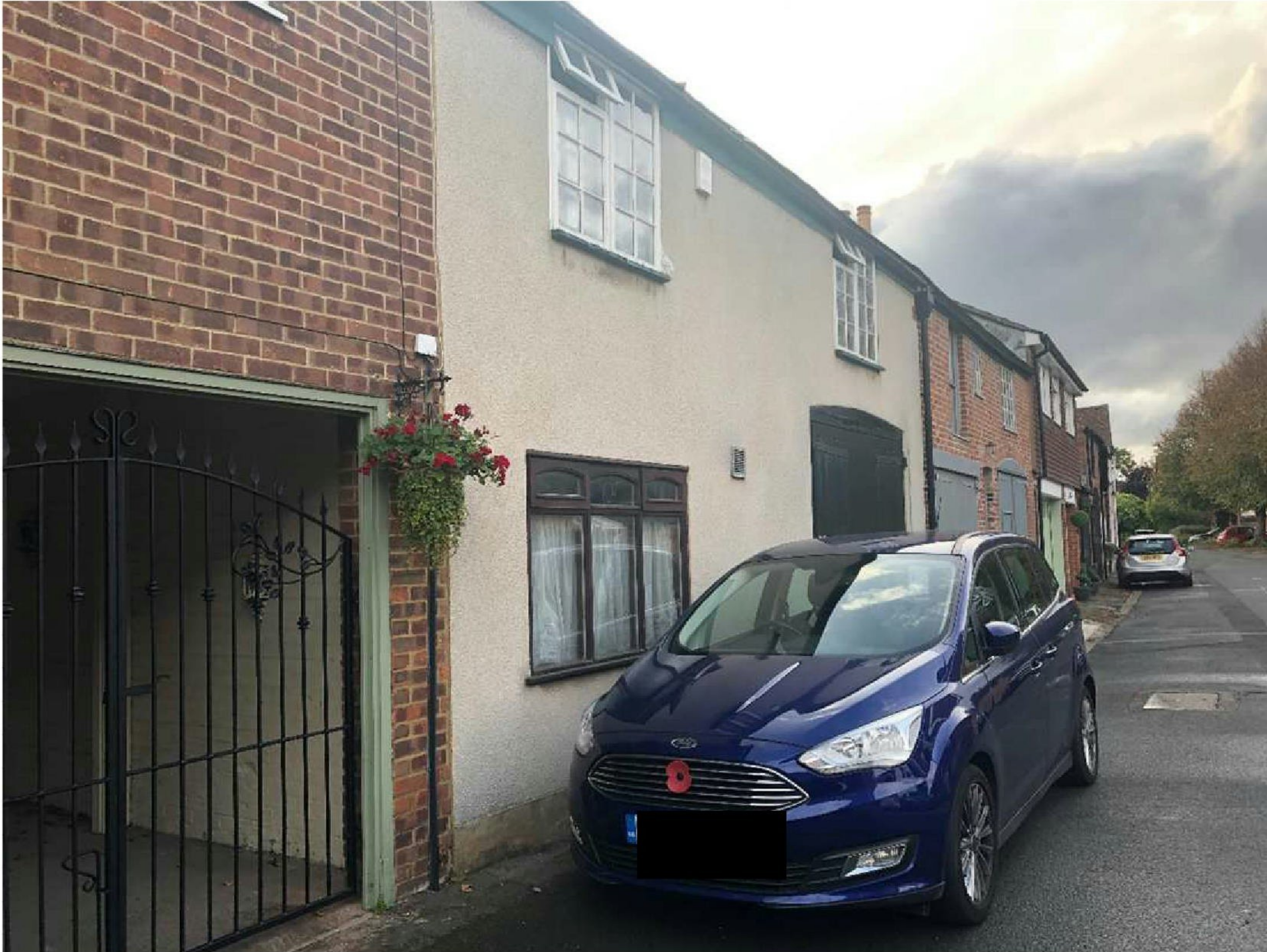
front (north) elevation showing 'modern' kitchen window (to be replaced)
