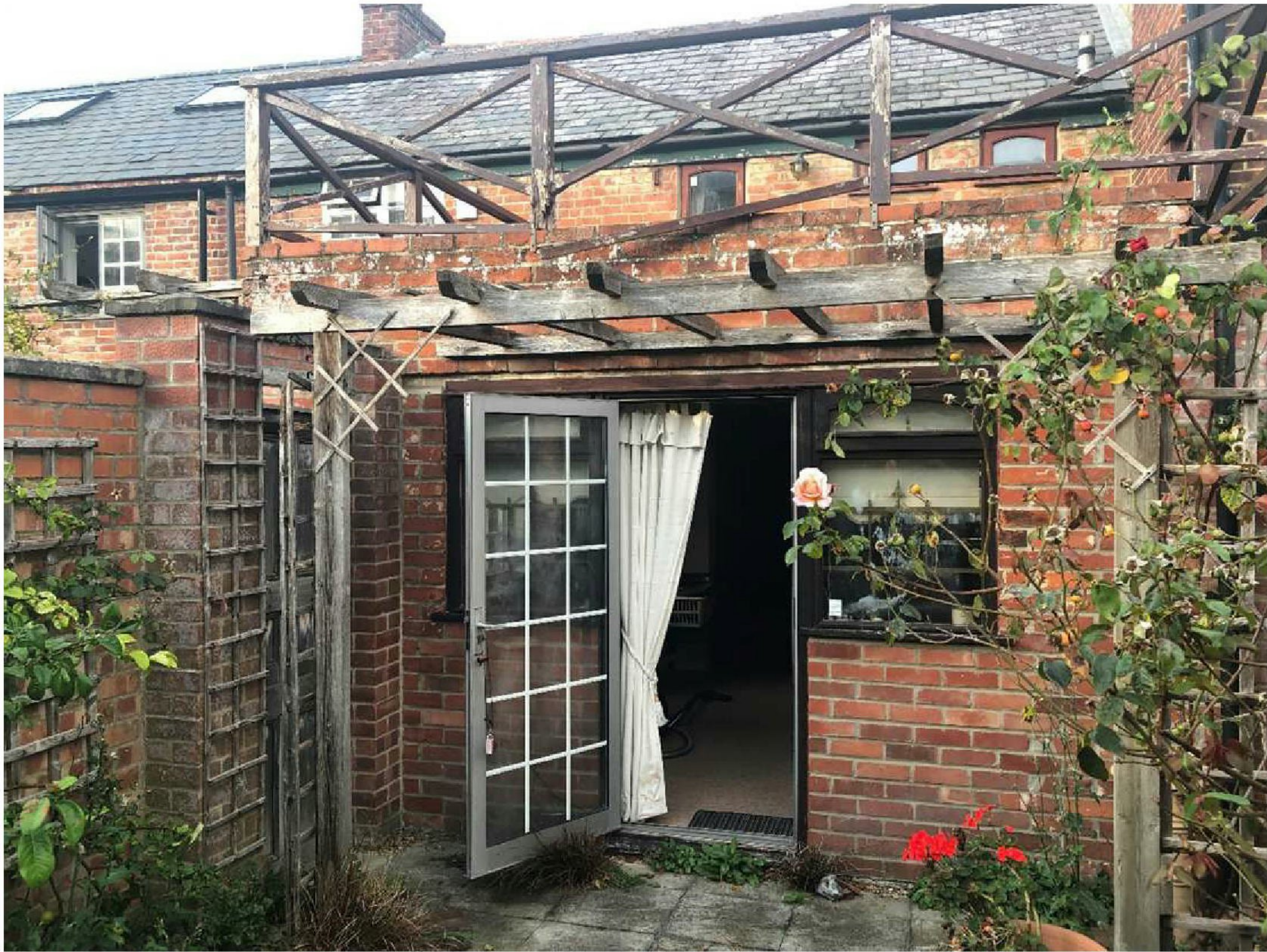
lounge viewed from rear courtyard garden
