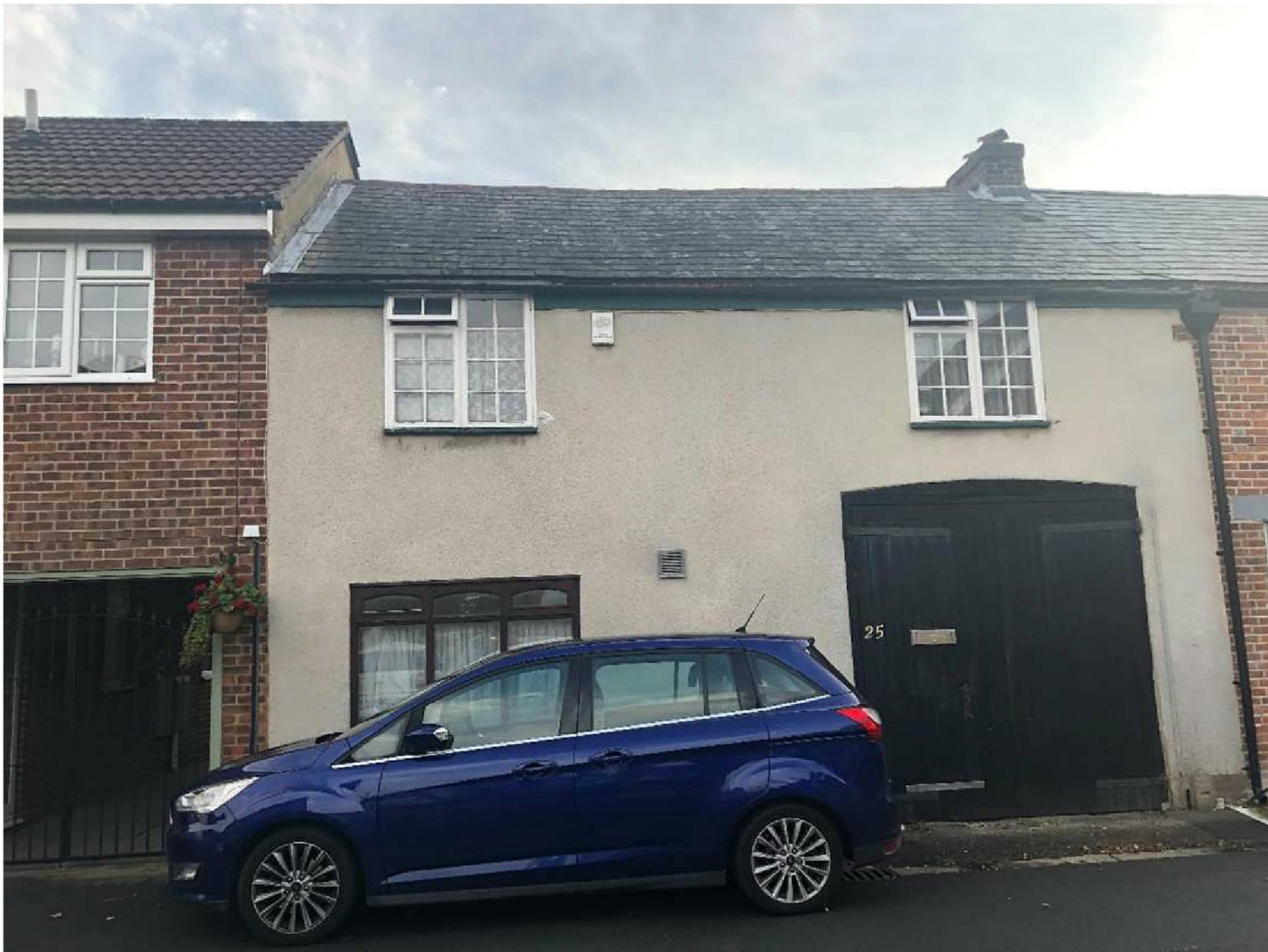
front elevation showing old coach entrance doors
