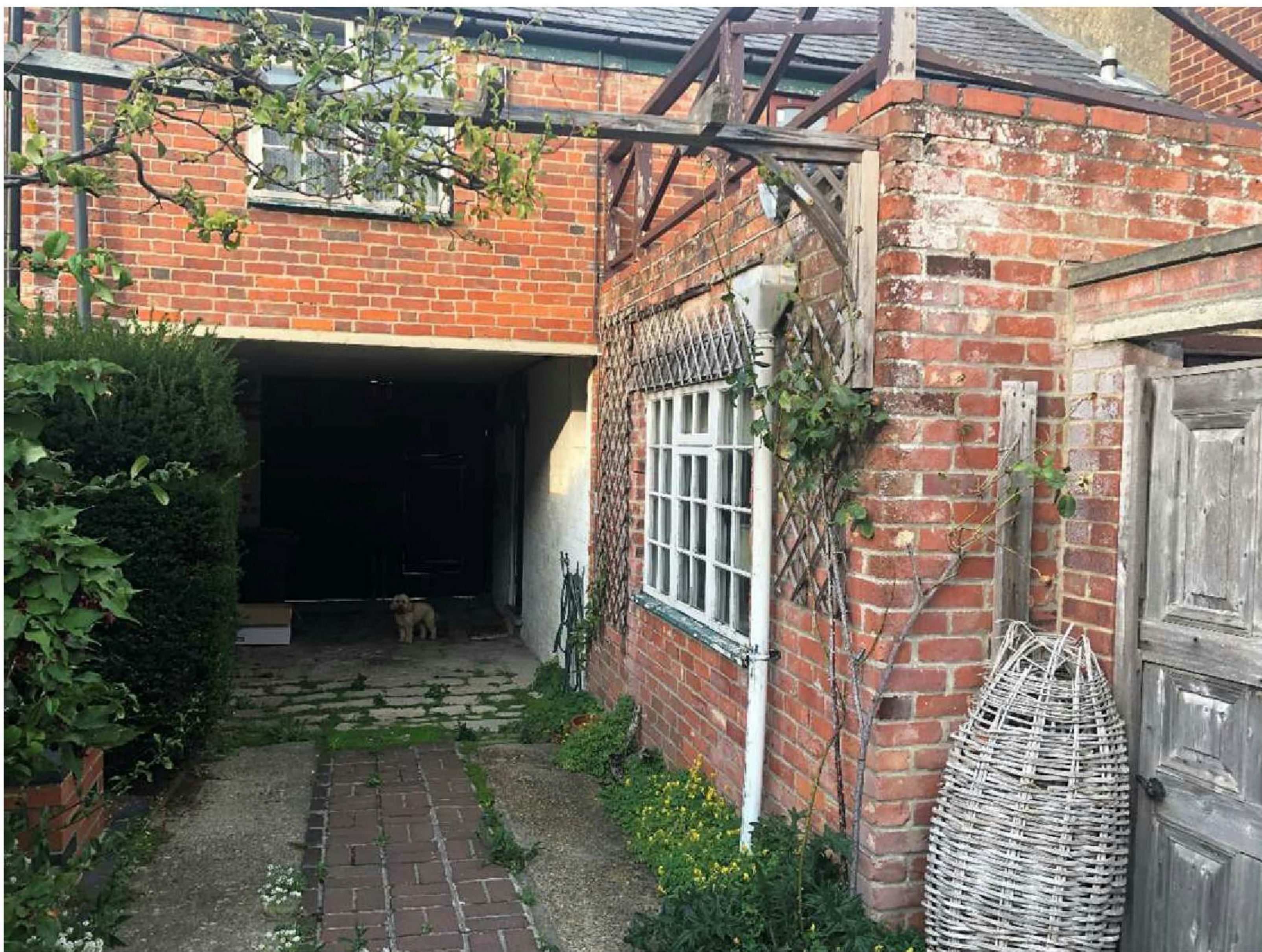
Undercroft viewed from rear driveway
