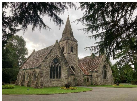
View from main approach
