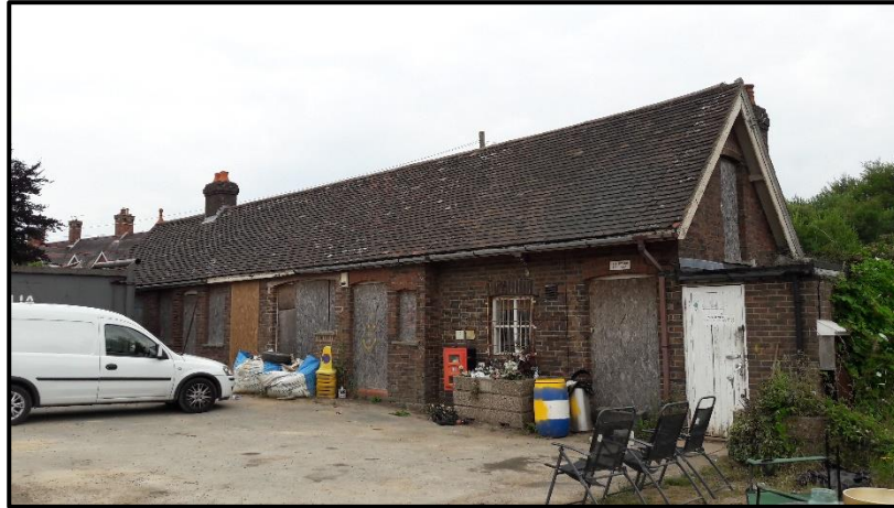
Photo 4.2: Building 1, facing north.
