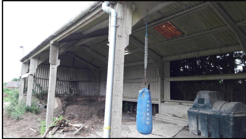
Photo 4.4: Building 2 – south-eastern section.
