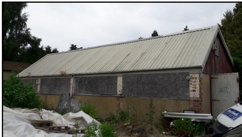
Photo 4.5: Building 3, looking west.
